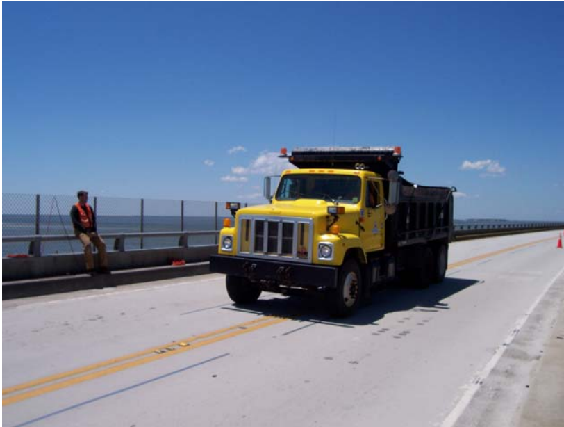
Figure 7. Truck positioned with right wheel over Girder No. 3 (looking north).
