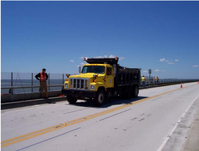
Figure 6. Truck positioned with left wheel over Girder No. 3 (looking north).
