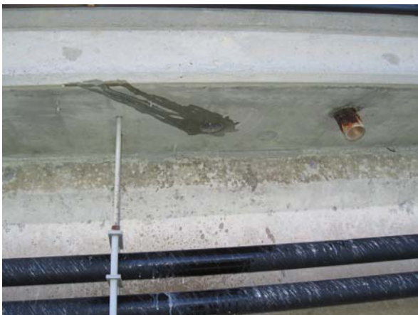
Span 161-162, Midspan deck core
