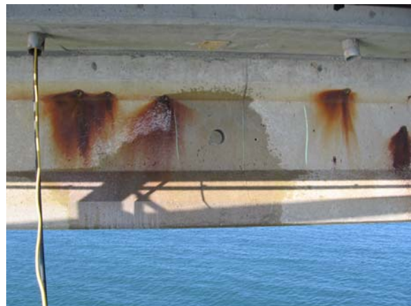
Span 131-132, Girder #4 core
