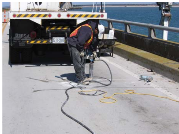
Span 161-162, South deck core
