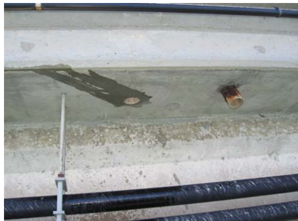
Span 161-162, Midspan deck core
