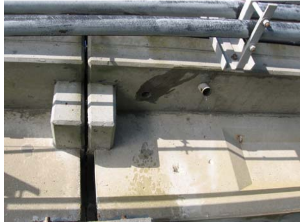
Span 131-132, South deck core
