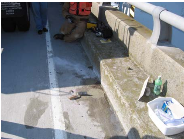
Span 149-150, South deck core
