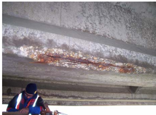
Span 160-161; SP & ES on Girder #2, East side,
