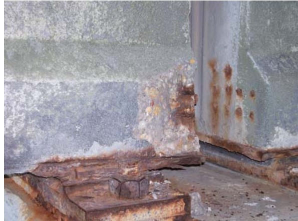
Span 134-135; SP at girder #2, East side, North
