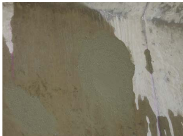
Span 149-150, Girder #2 core
