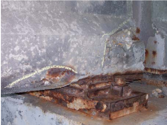
Span 134-135; SP & ES at Grder #2, East side,
