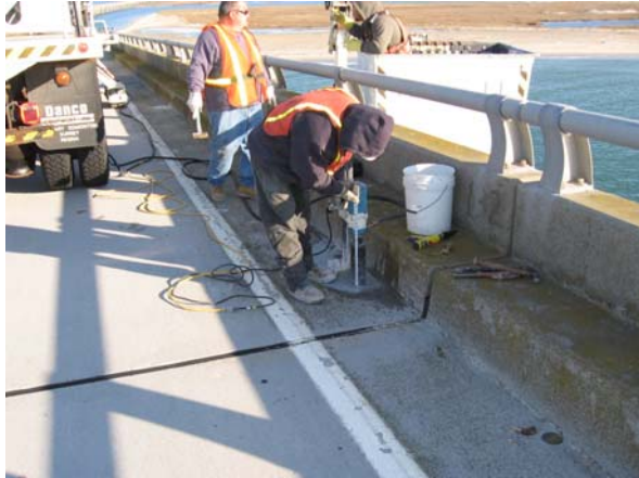
Span 131-132, South deck core
