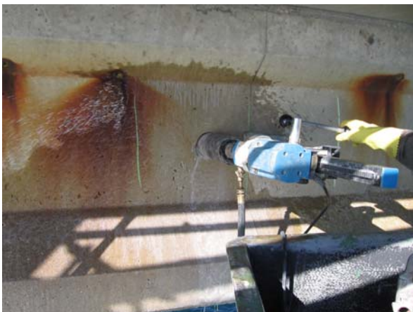
Span 131-132, Girder #4 core
