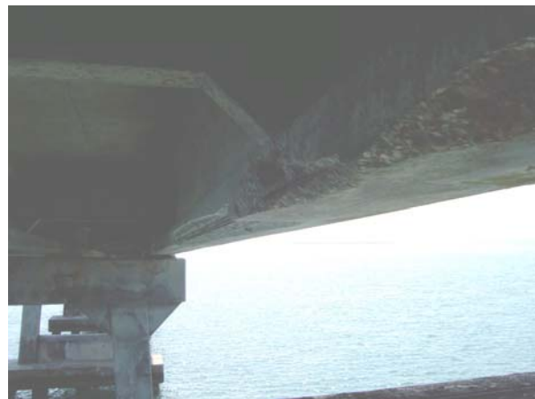
Span 161-162; SP & ESx5 on Girder #4, East
