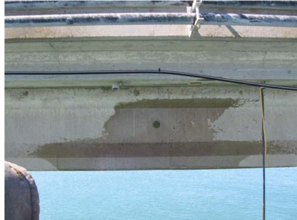
Span 129-130, Girder #4 core
