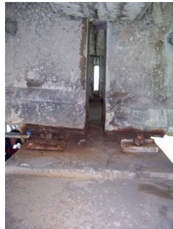
Span 139-140; Overall shot of Grder bearings @
