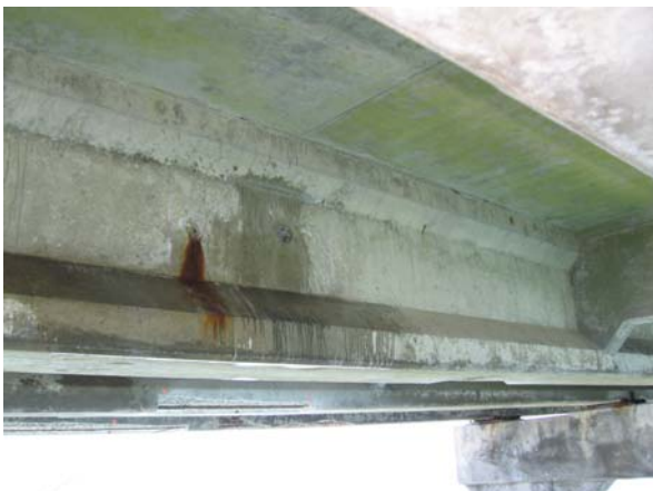
Span 161-162, Girder #3 core
