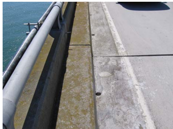
Span 129-130, South deck core
