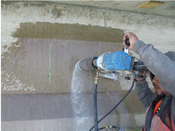
Span 129-130, Girder #4 core
