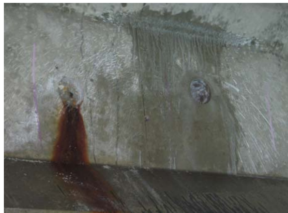
Span 161-162, Girder #3 core
