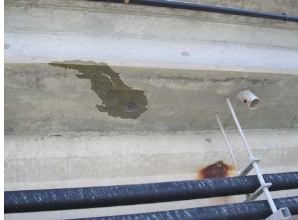
Span 149-150, South deck core
