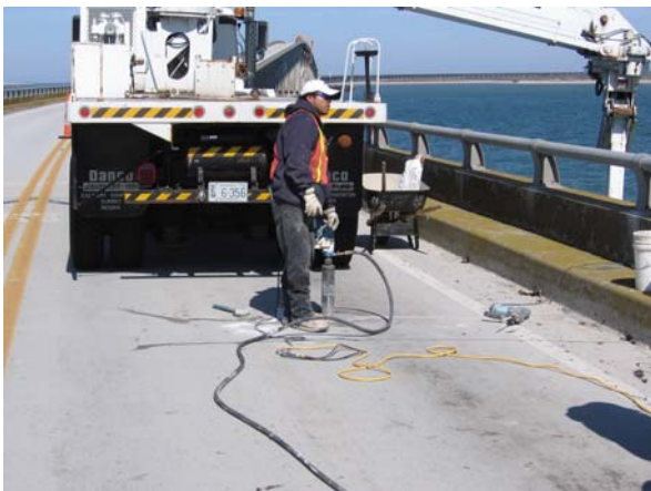
Span 161-162, South deck core
