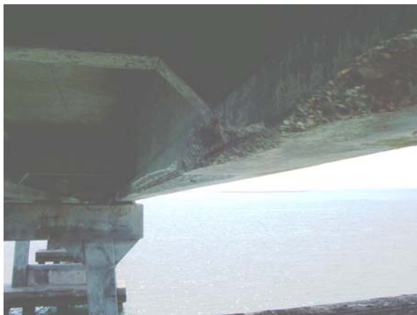
Span 161-162; SP & ESx5 on Girder #4, East
