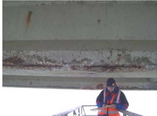
Span 162-163; SP & ES on Girder #3, East side,
