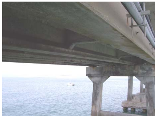
Span 162-163; Overall of span
