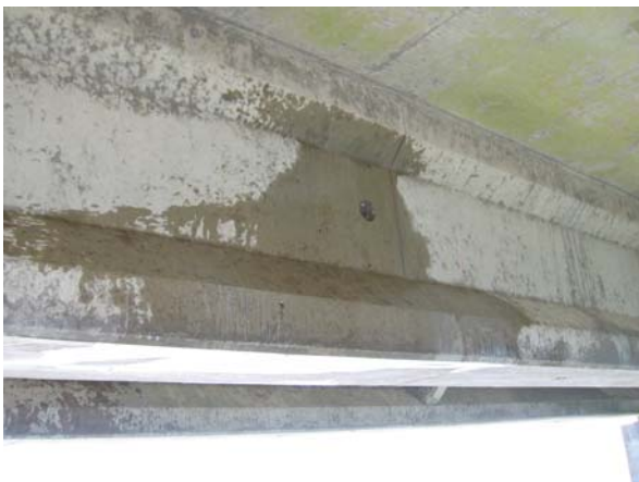
Span 149-150, Girder #2 core
