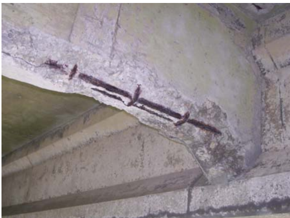
Span 160-161; SP & ER on South diaphragm,
