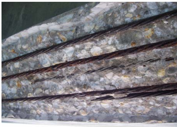
Span 161-162; SP & ESx5 on Girder #4, East
