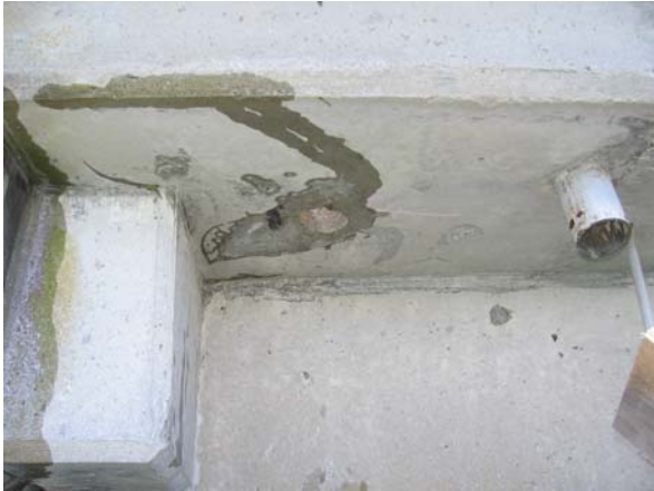
Span 149-150, South deck core
