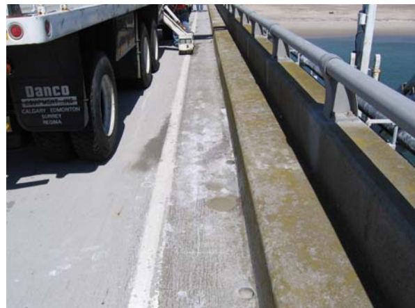
Span 129-130, Midspan deck core
