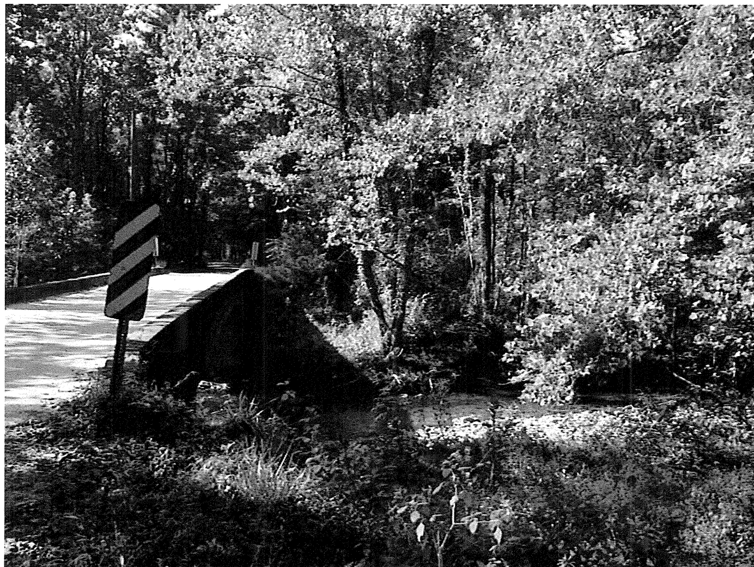
Looking South along NC 90 (Creek flow right to left)
