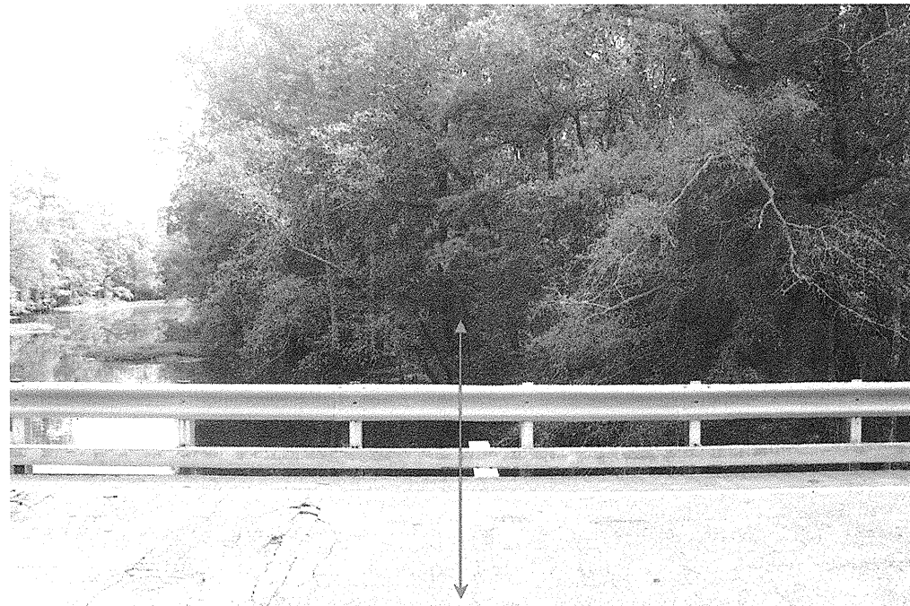
Photograph No. 4: Cross-section view of Bent 2, looking south.
