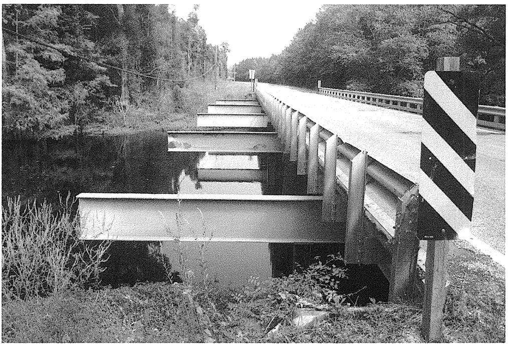
Photograph No. 7: North side of bridge, looking east.
