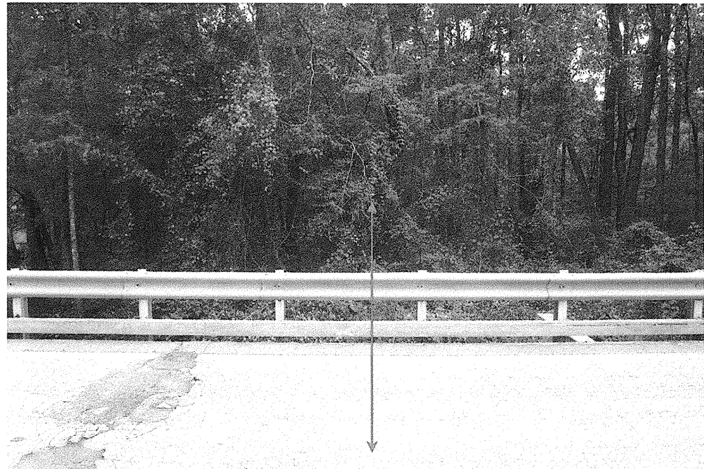
Photograph No. 3: Cross-section view of Bent 1, looking south.
