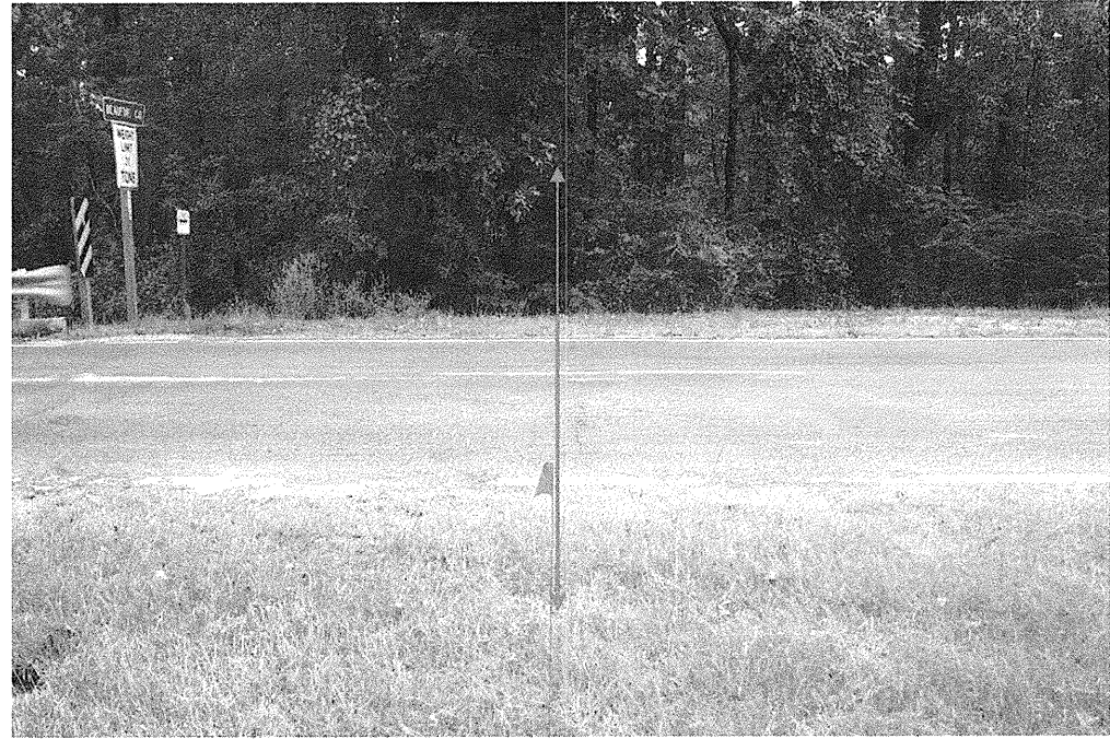
Photograph No. 2: Cross-section view of End Bent 1, looking south.
