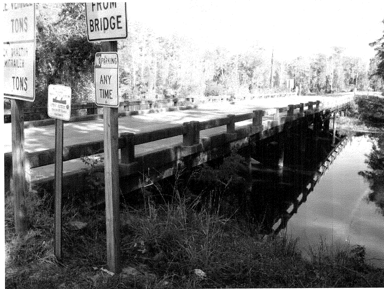
View Looking Northeast Toward End Bent 2
