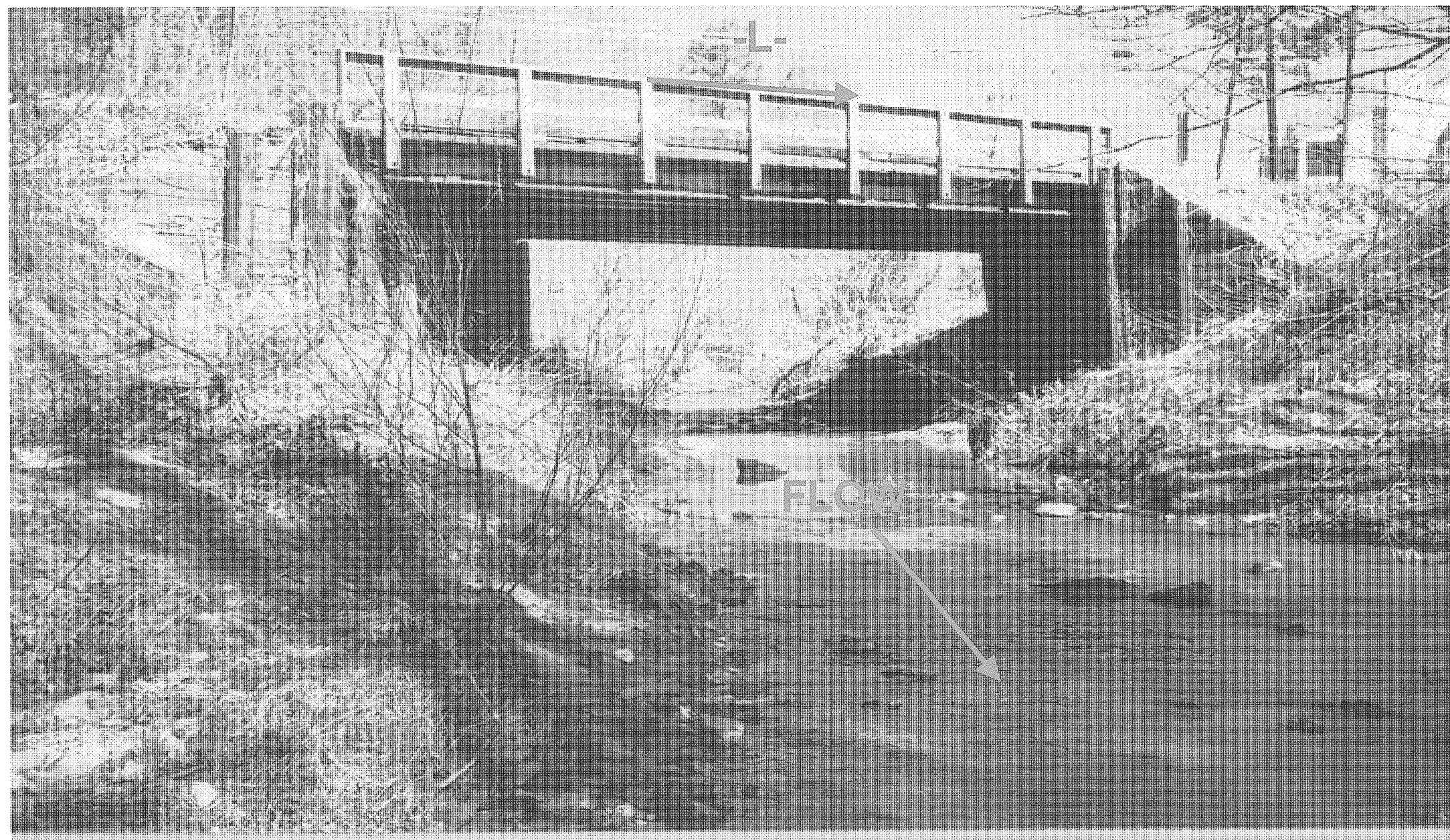
BRIDGE NO. 73 OVER BULL RUN CREEK ON SR 1549 (MACKAY RD.)
