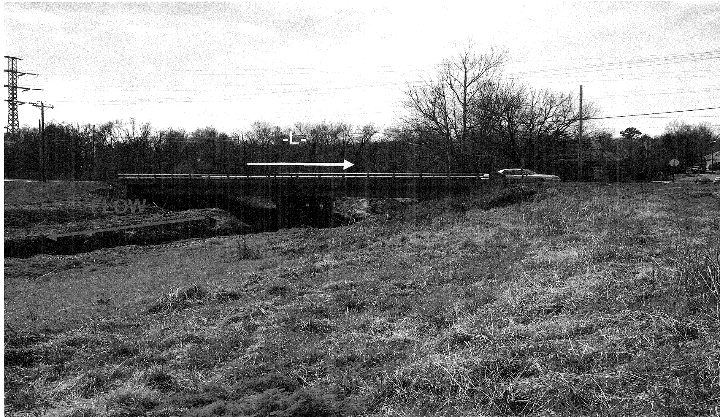
LOOKING SOUTHWEST TOWARD END BENT 1
