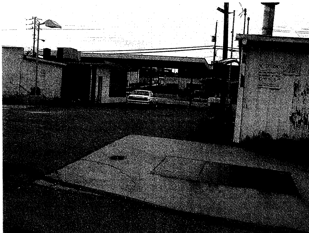
Oil/Water separator. Service station in background
