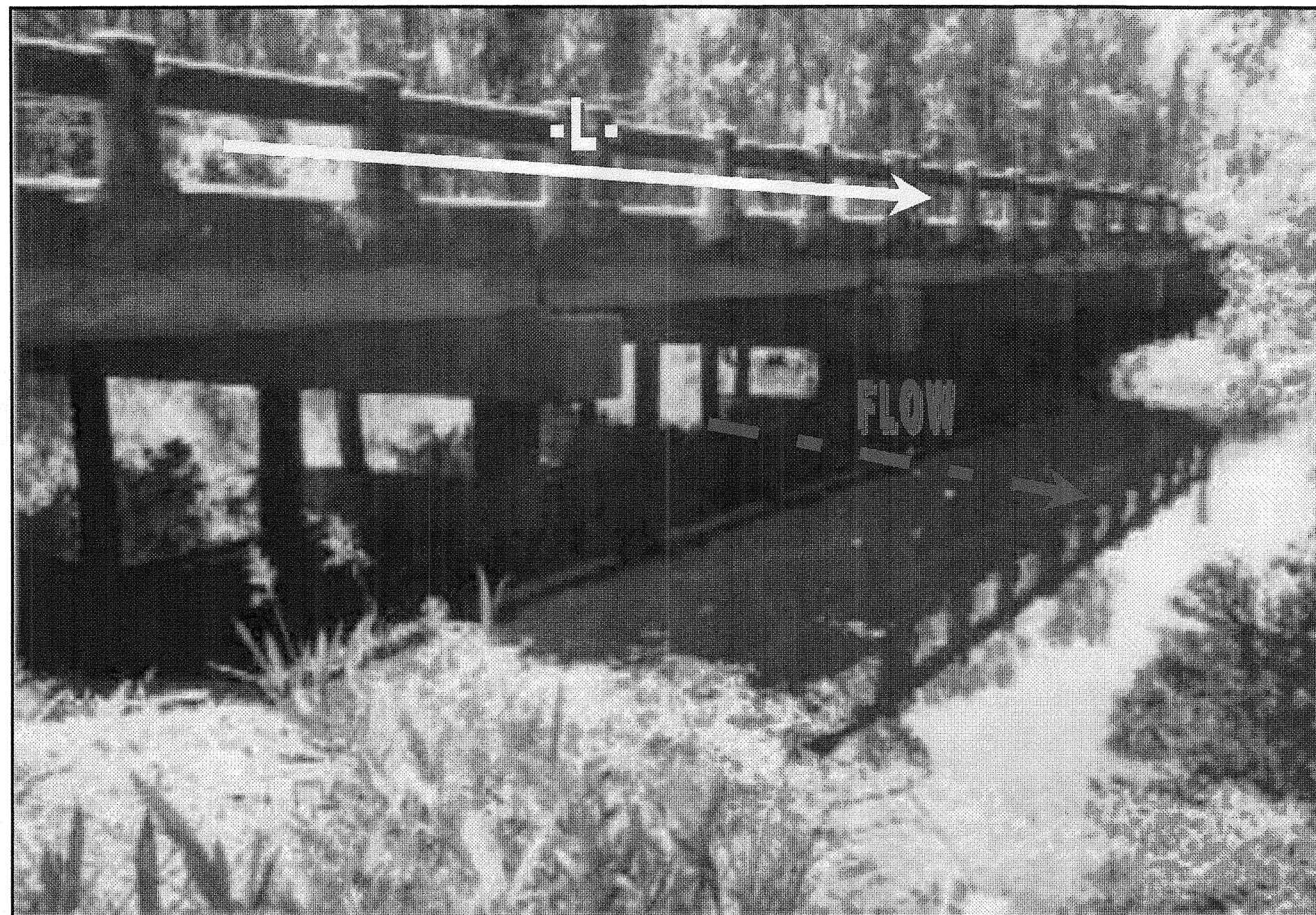
BRIDGE NO. 98 ON SR 1246 (BUTLER ISLAND RD.) OVER BIG SWAMP
