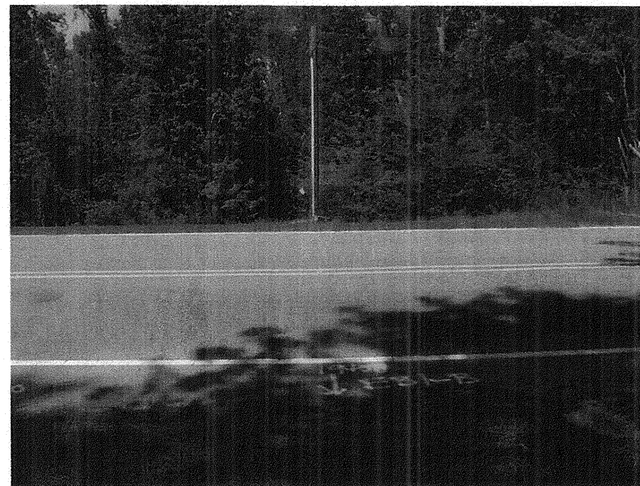
Photograph No. 3: This photograph was taken from the right side of the -EL- alignment, looking northeast, across proposed End Bent No.1.
