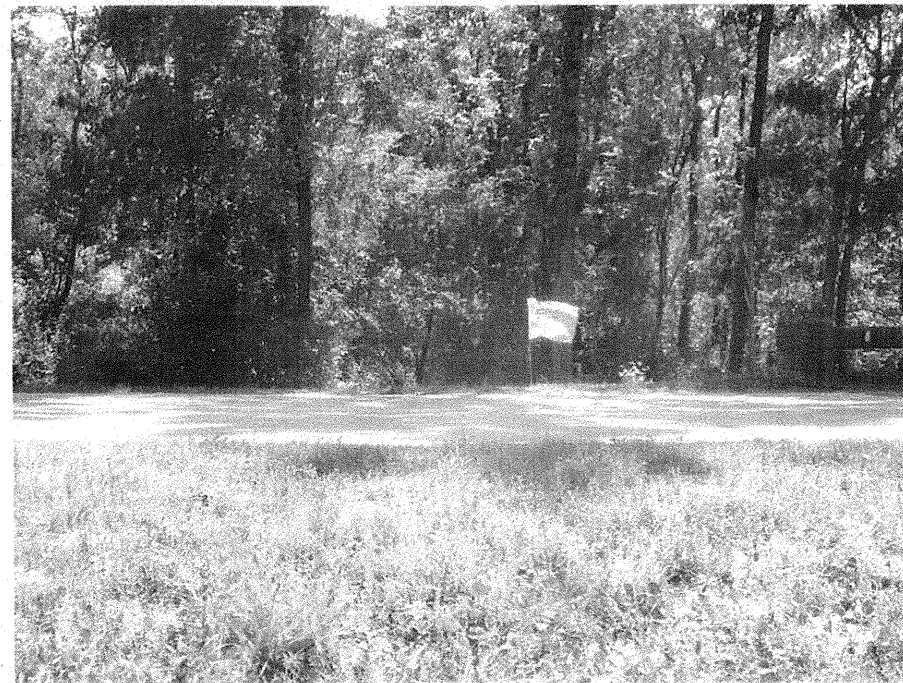
Photograph No. 10: This photograph was taken from the left side of the -EL- alignment, looking southwest, across proposed End Bent No.2.
