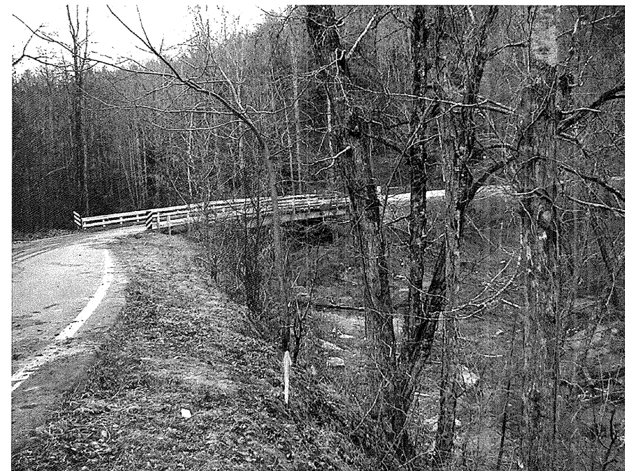
Looking along Temporary Shoring Alignment
