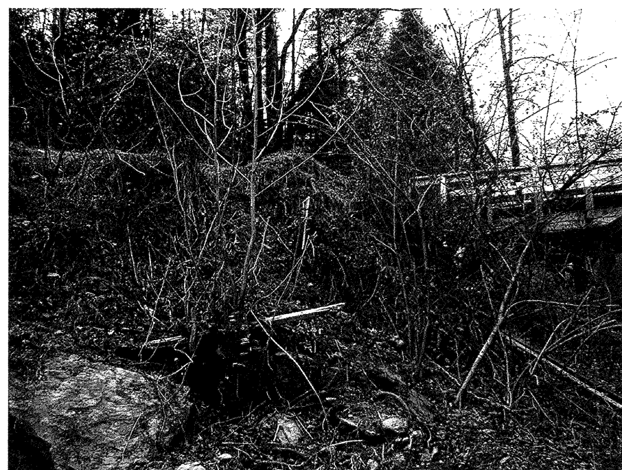
Looking from Corner of Retaining Wall toward TS-2
