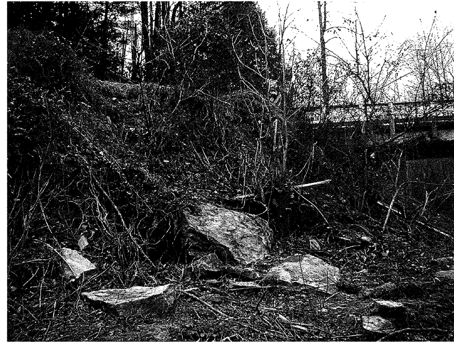
Looking Right to Left along End Bent-1
