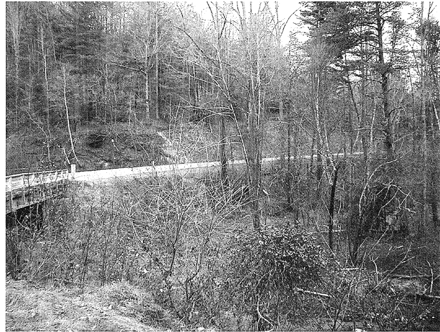
Looking Increasing Station along -L-
