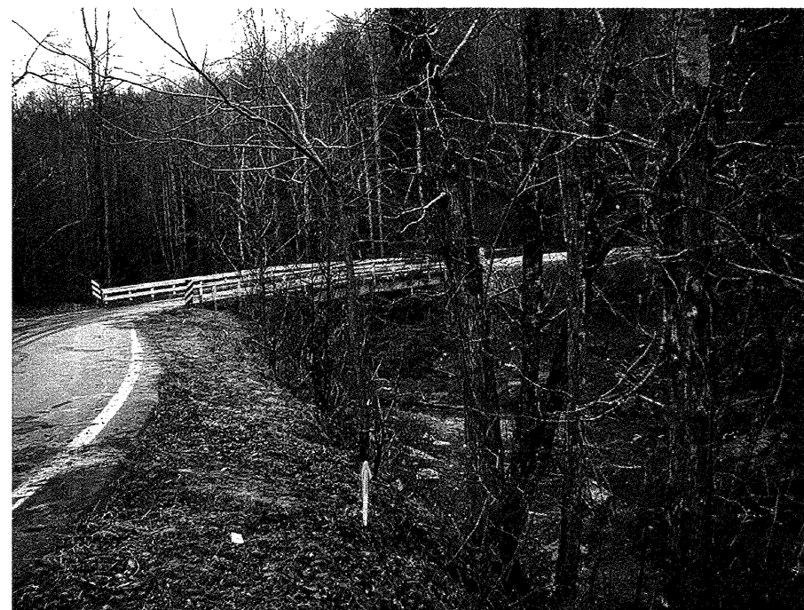
Looking from Beginning of Retaining Wall toward EB1-B
