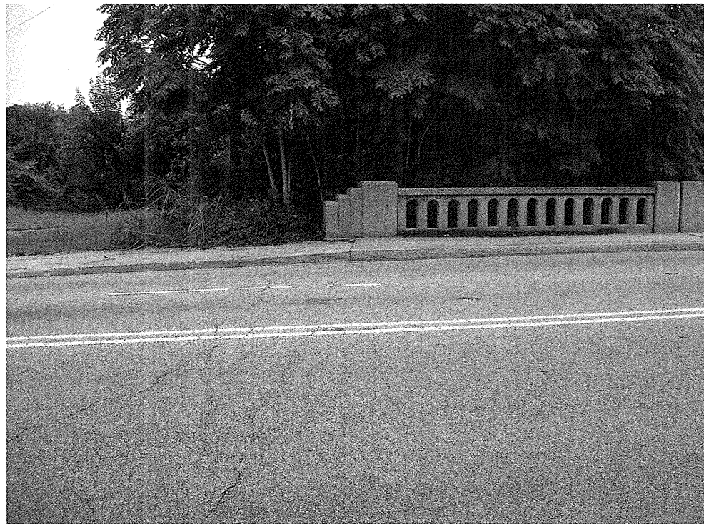
VIEW LOOKING NORTHEAST ALONG BENT - 1
