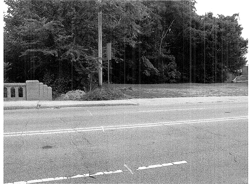
VIEW LOOKING NORTHEAST ALONG BENT - 2
