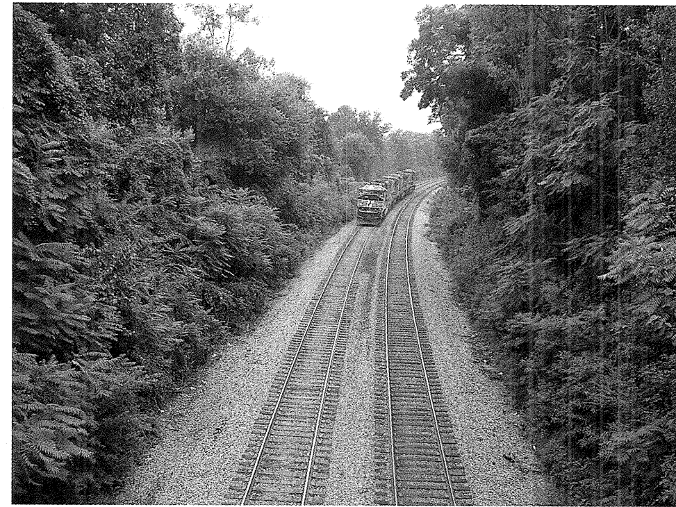
VIEW LOOKING NORTHEAST ALONG NSRR
