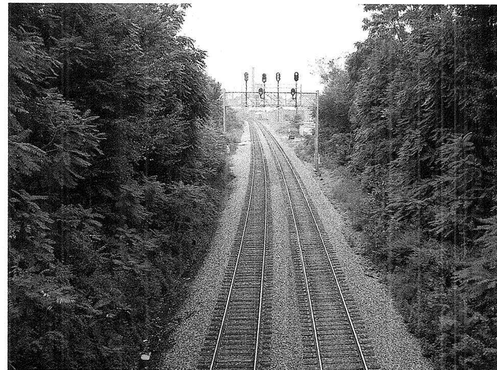
VIEW LOOKING SOUTHWEST ALONG NSRR
