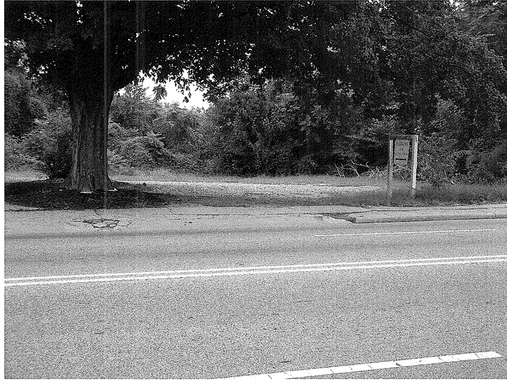
VIEW LOOKING NORTHEAST ALONG END BENT - 1
