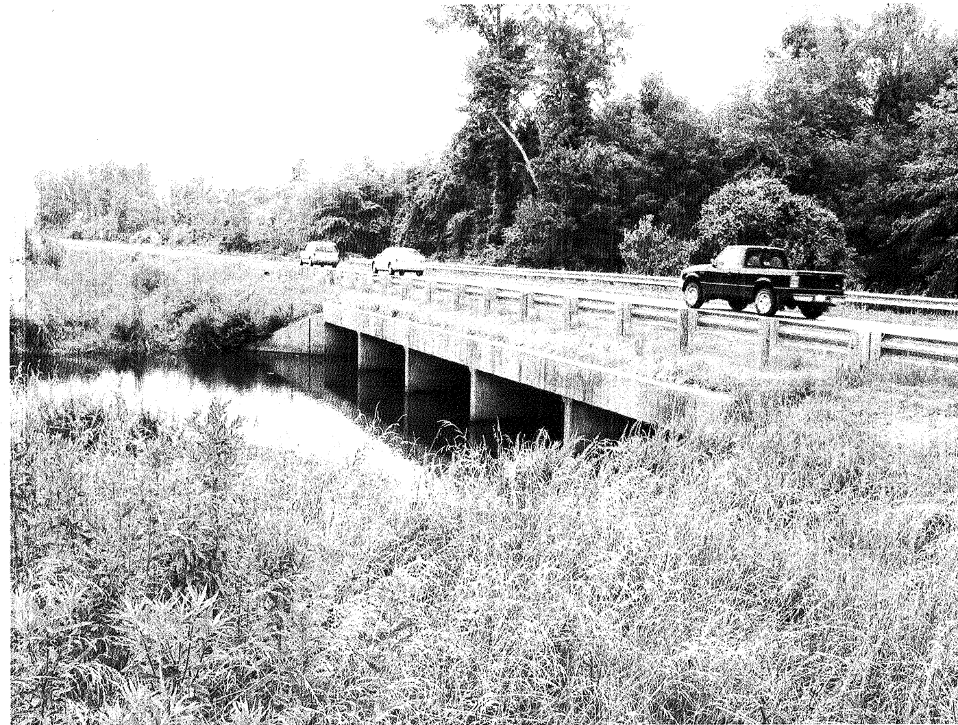
Looking south towards End Bent 1
