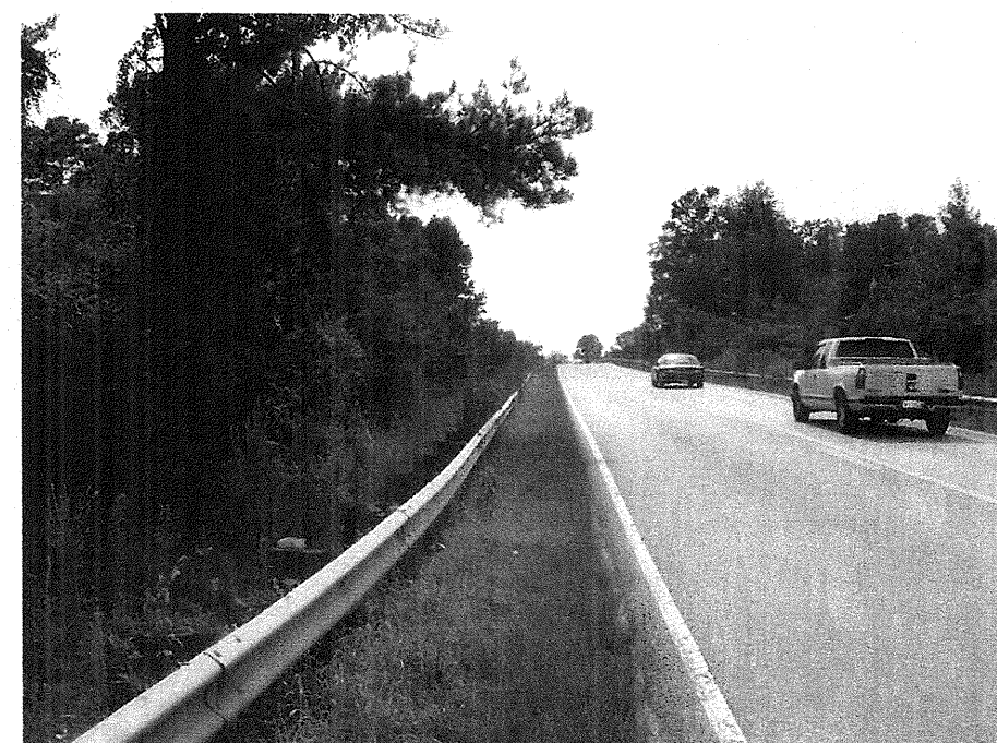
Photograph No. 16: This photograph was taken from existing NC 210, looking west, toward the existing bridge over the Northeast Cape Fear River.
