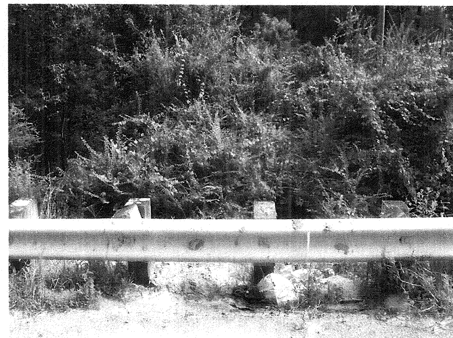
Photograph No. 12: This photograph was taken from the existing bridge, left of the -L- alignment, looking south, across proposed Interior Bent No. 7.
