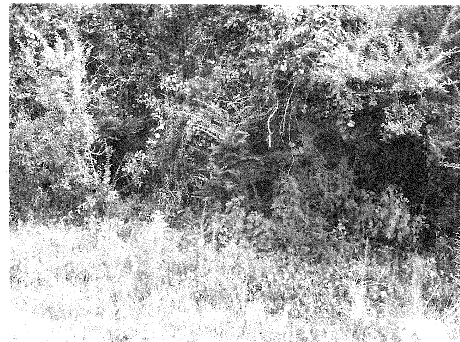
Photograph No. 15: This photograph was taken from the existing bridge, left of the -L- alignment, looking south, across proposed End Bent No. 2.
