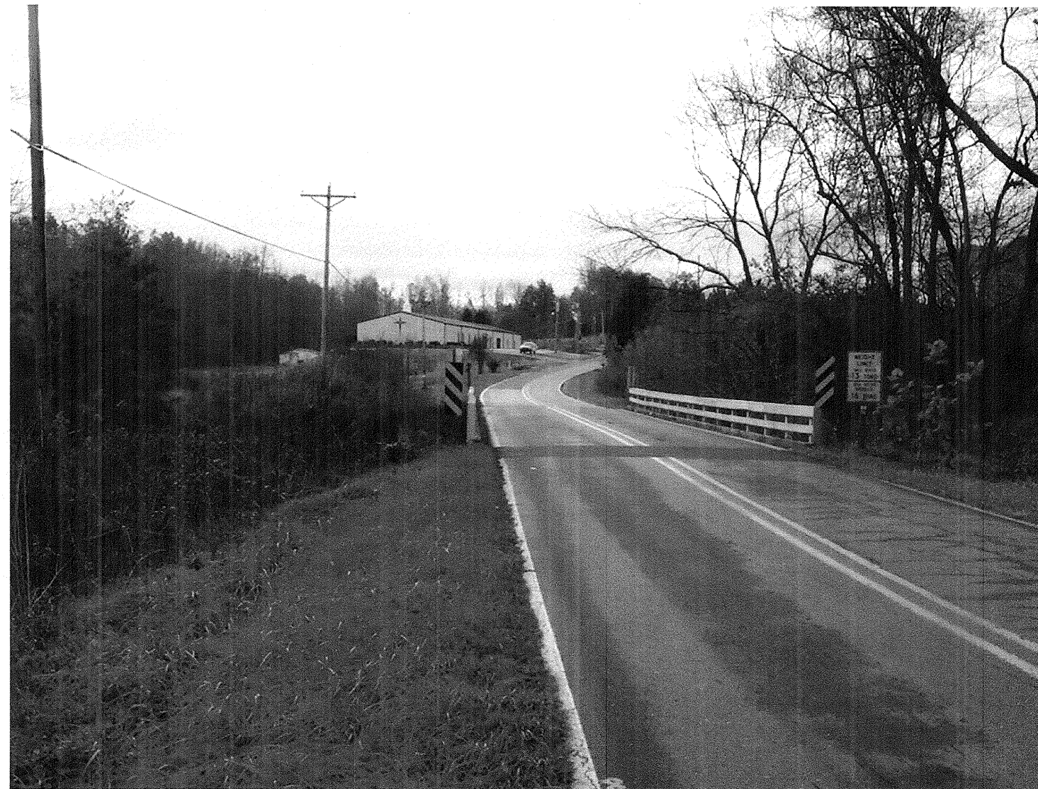
Looking South along SR 1521 (Creek flow right to left)
