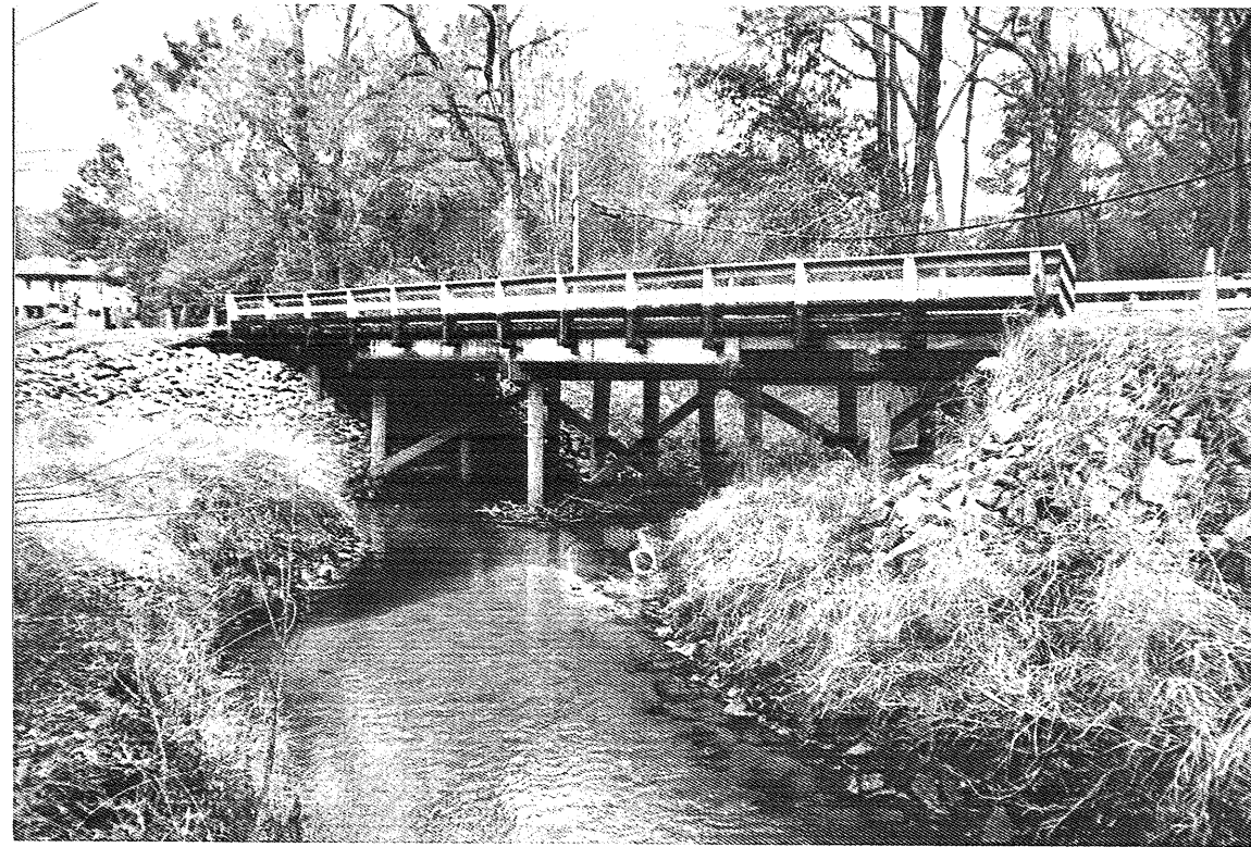
Photograph No. 1: Looking northwest, downstream to the existing bridge.
