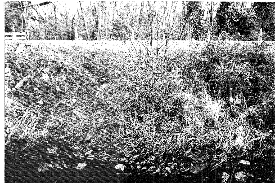
Photograph No. 7: Looking north along bent 3, located just right of the red traverse marker BL-3.
