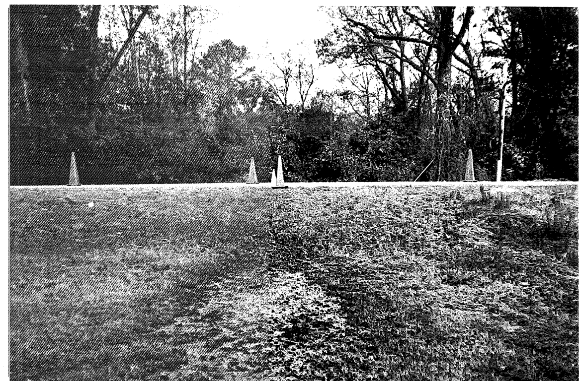
Photograph No. 4: Looking north along end bent 1.
