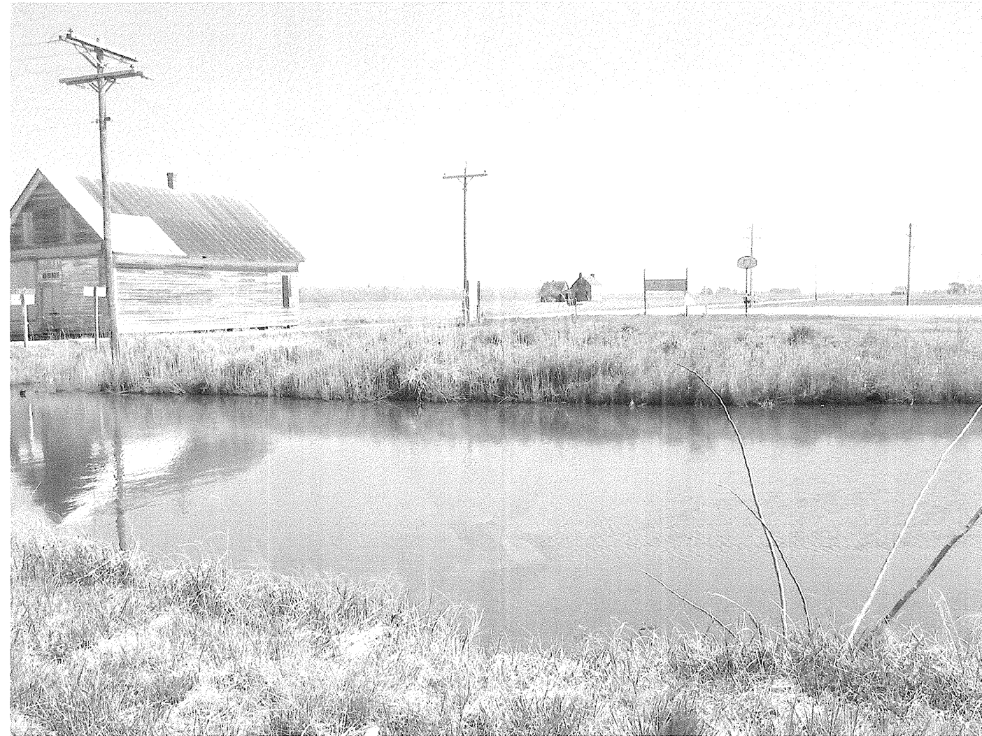
Looking east towards End Bent 2
