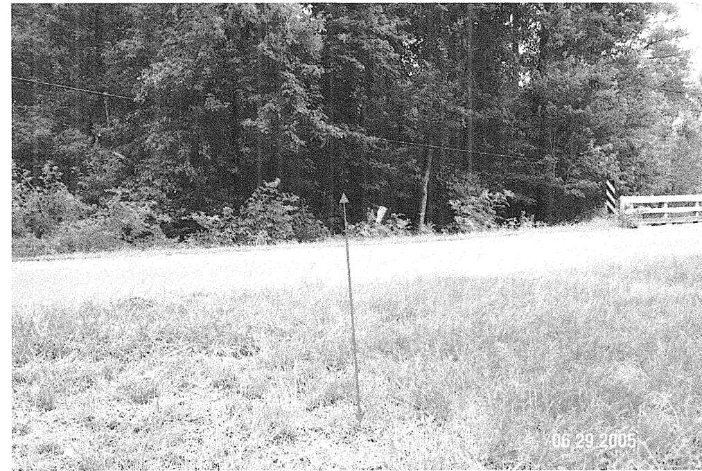
Photograph No. 4: Cross-section view of End Bent 2, looking east.
