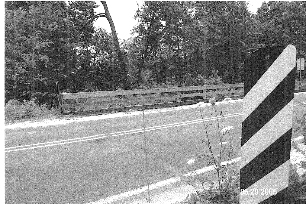
Photograph No. 3: Cross-section view of Bent 1, looking west.
