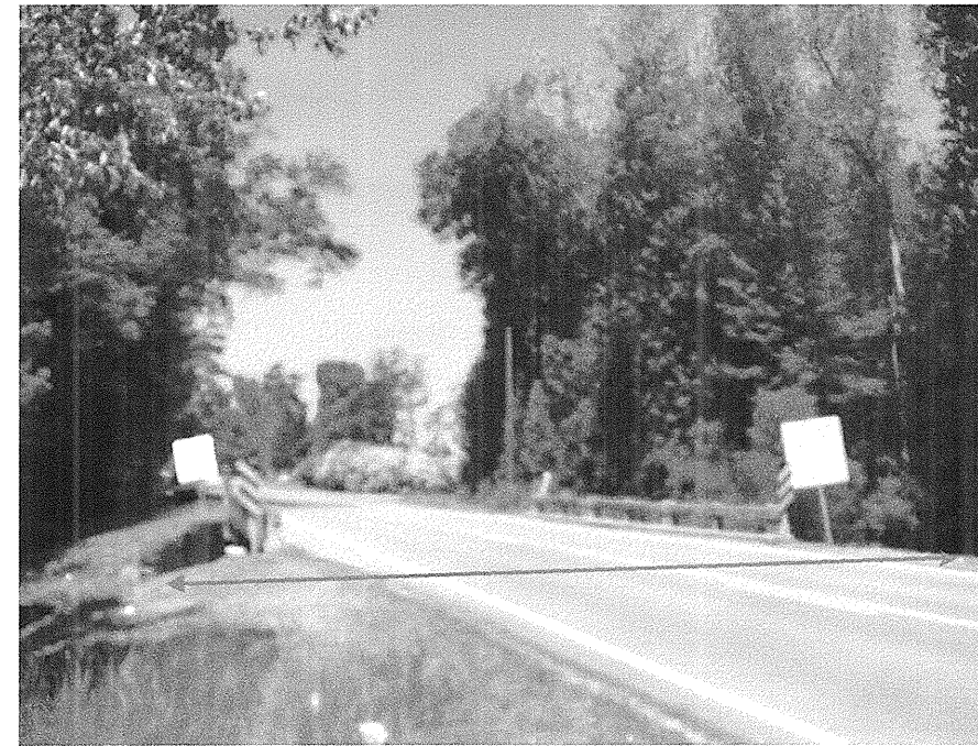
Photograph No. 3: Cross-section view of End Bent 2, looking west.
