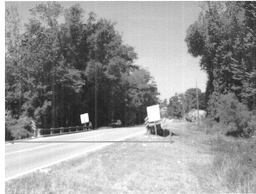
Photograph No. 4: Cross-section view of End Bent 2, looking west.
