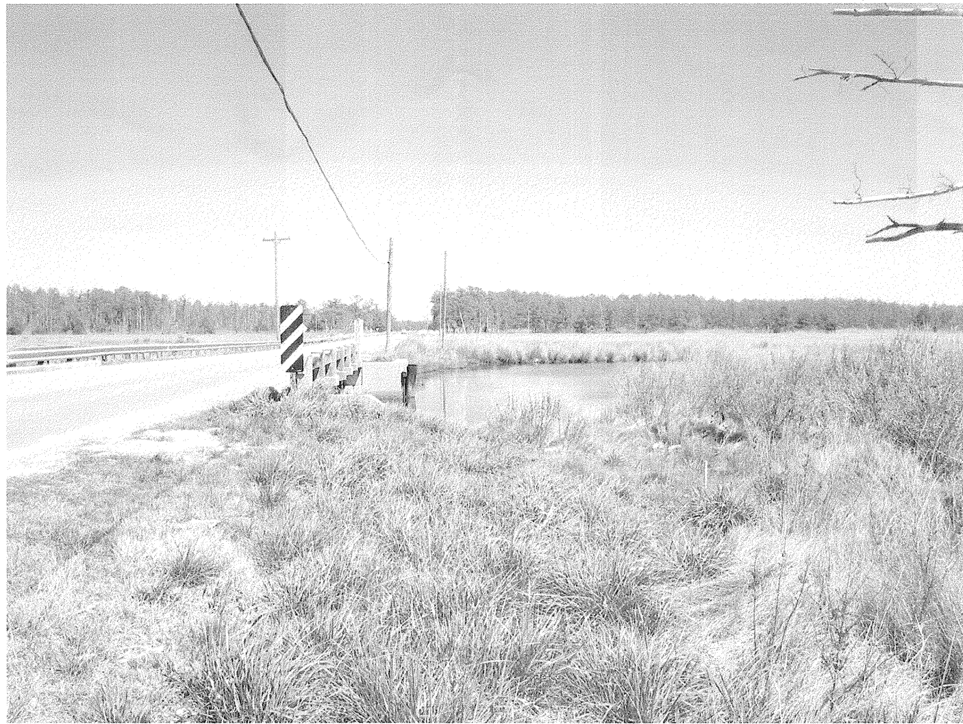
Looking north towards End Bent 2
