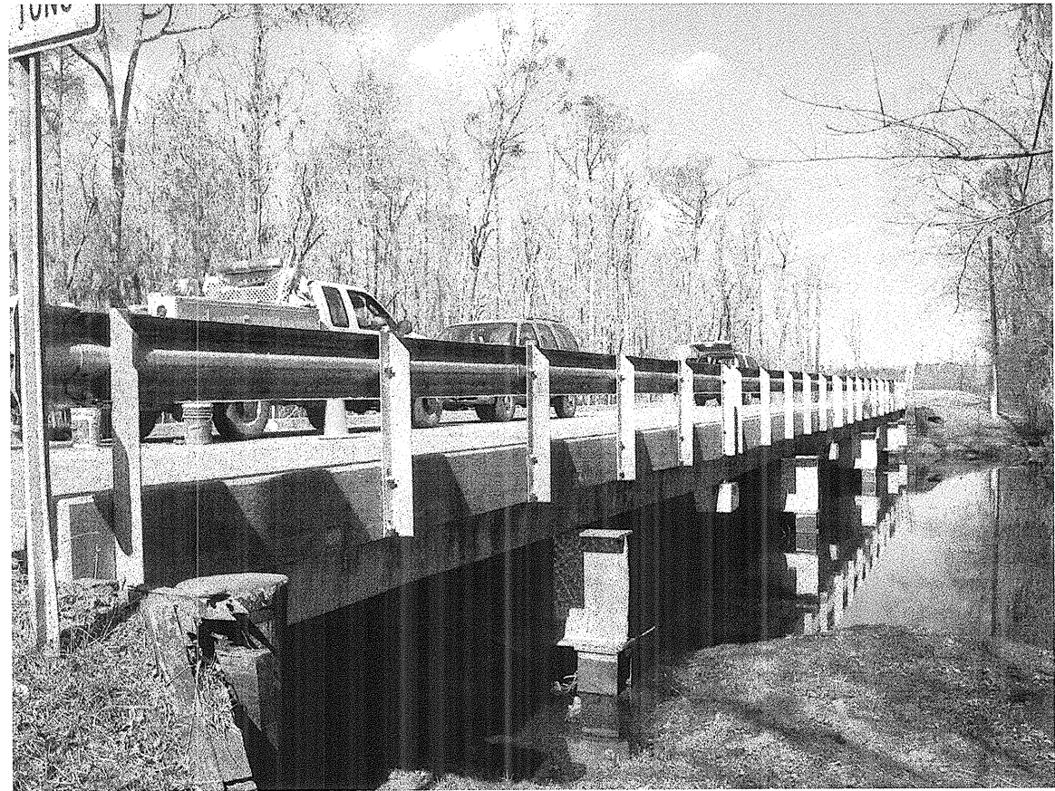
Looking North Towards End Bent 2
