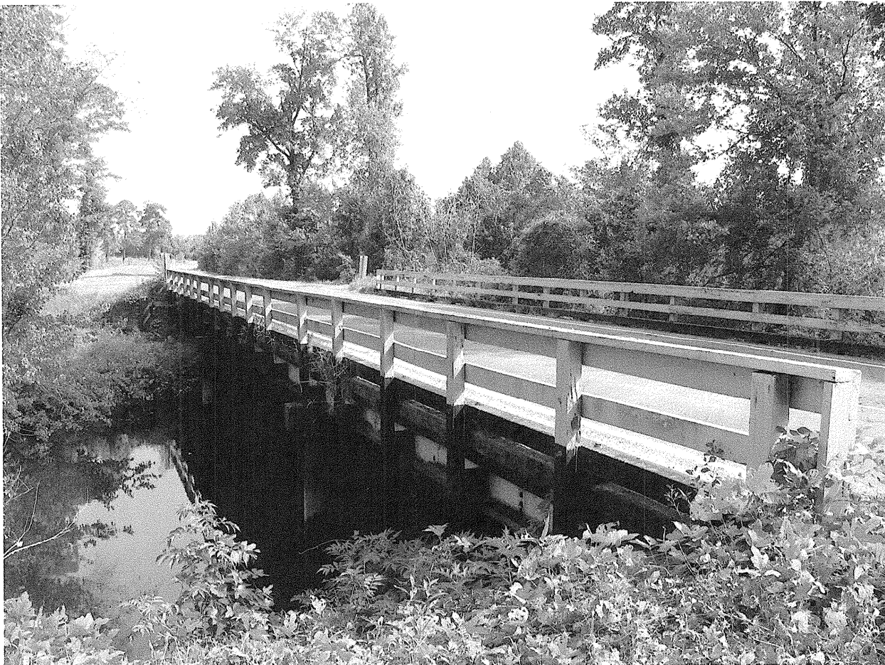
Looking north towards End Bent 2
