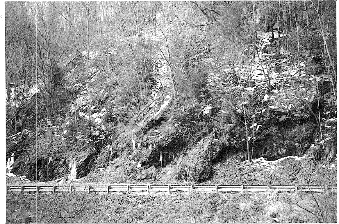
FIGURE 1: VIEW APPROXIMATE STATION 18+50 - 20+00
