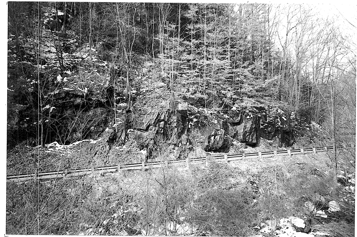
FIGURE 2: VIEW APPROXIMATE STATION 19+50 - 22+00
