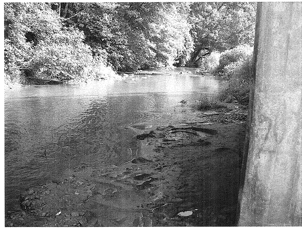
VIEW LOOKING NORTH ALONG BENT -1
