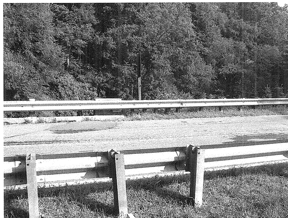
VIEW LOOKING NORTH ALONG END BENT - 1
