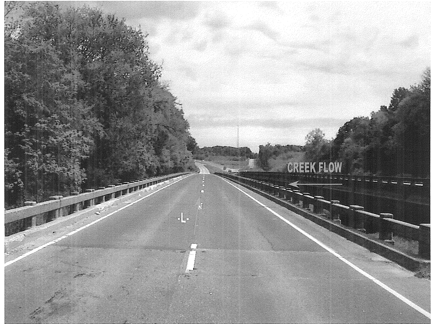
VIEW OF US 74 WBL BRIDGE LOOKING TOWARDS POLKTON
