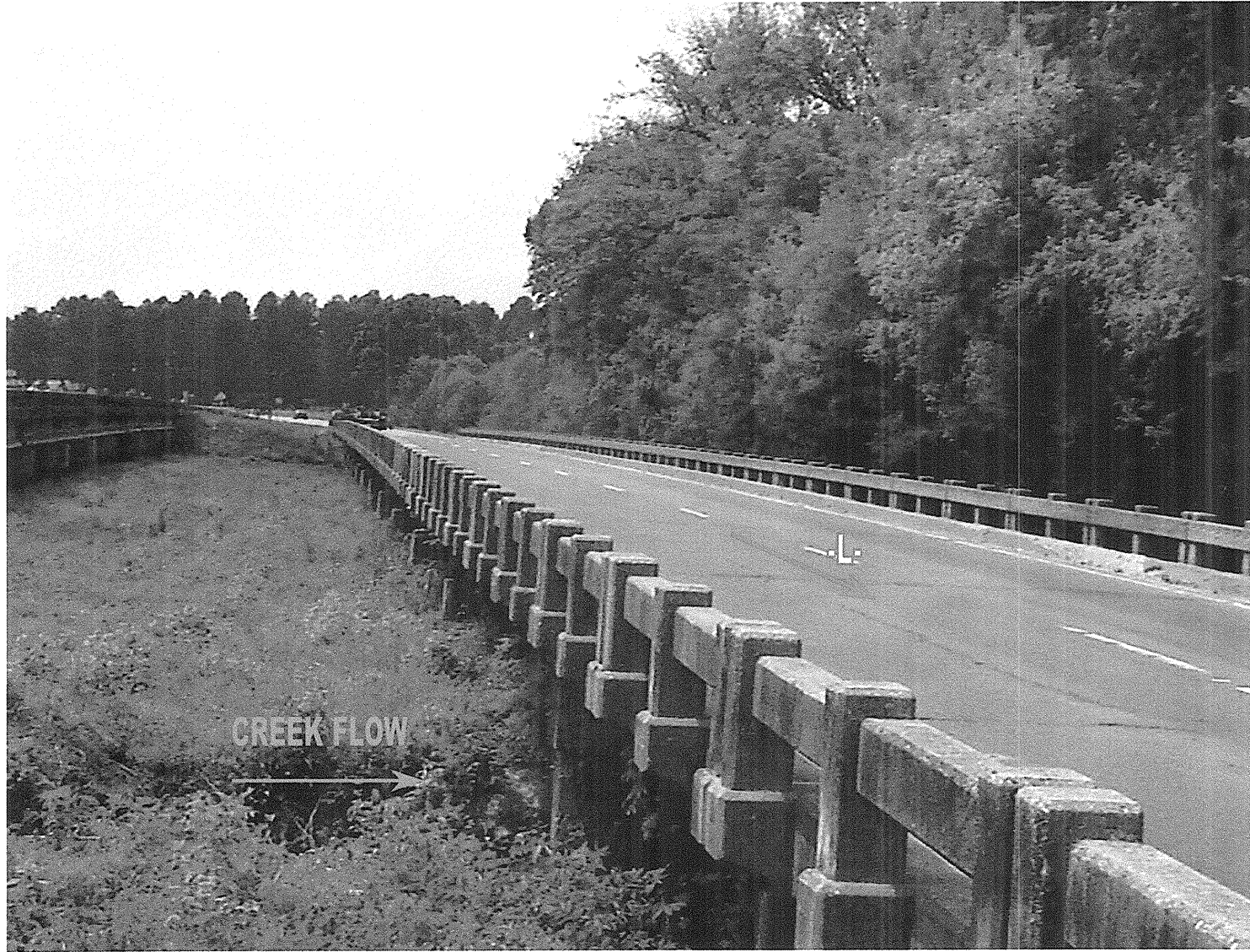
VIEW OF US 74 WBL BRIDGE LOOKING TOWARDS CHARLOTTE
