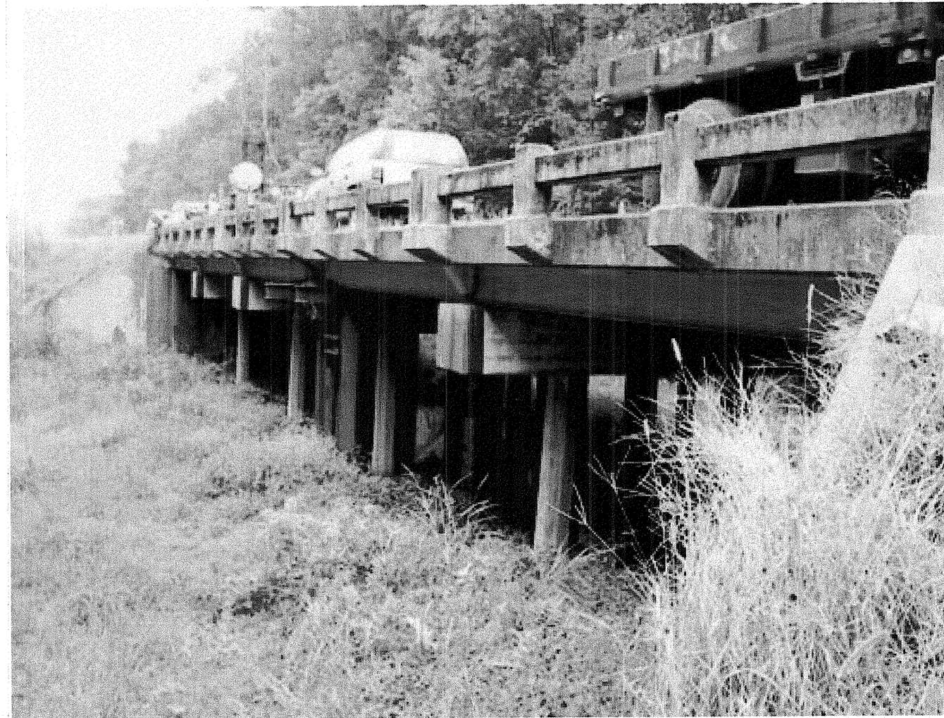
Looking North Towards End Bent 2
