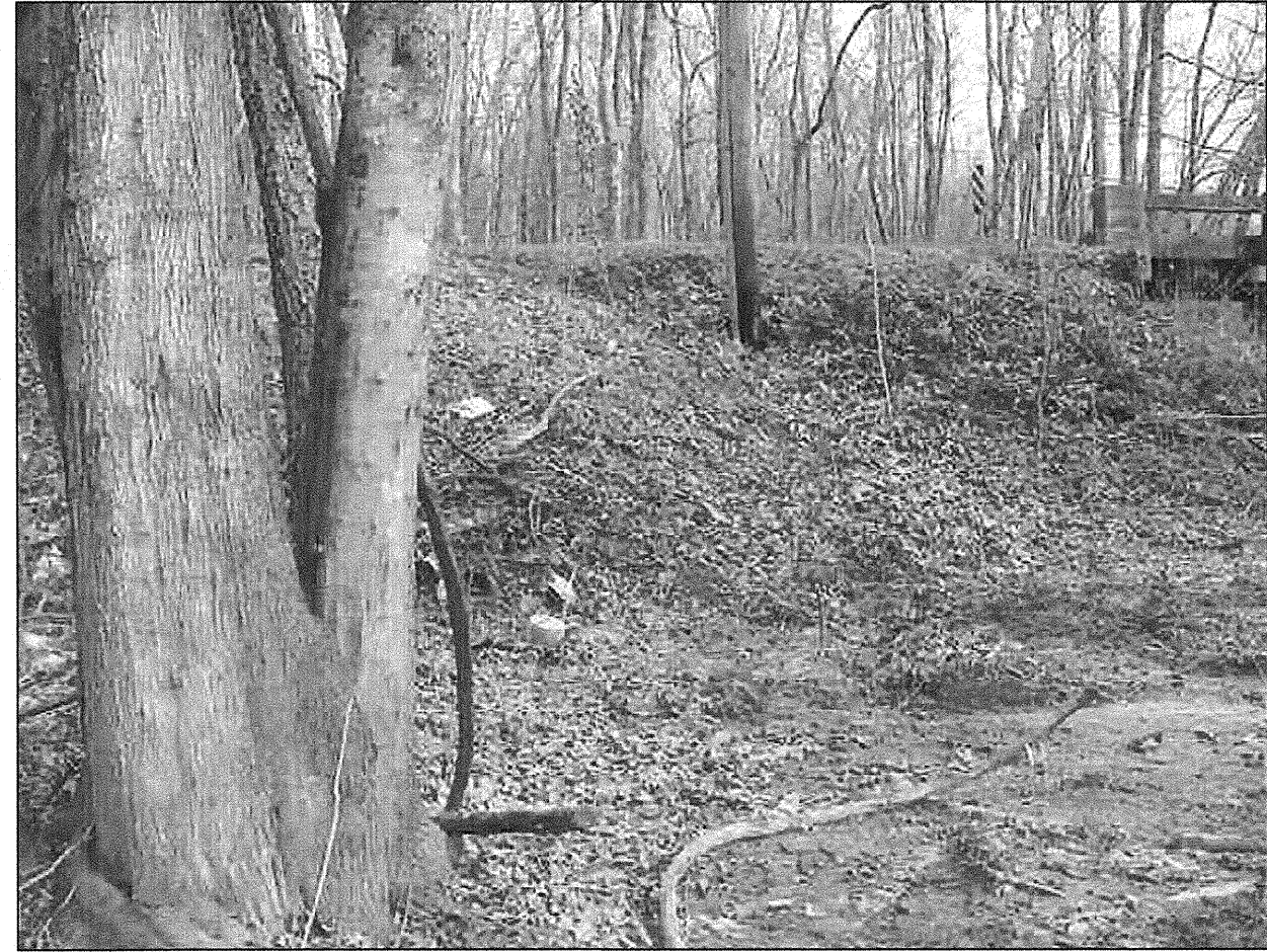
End Bent 2, looking from EB2A to EB2B.
