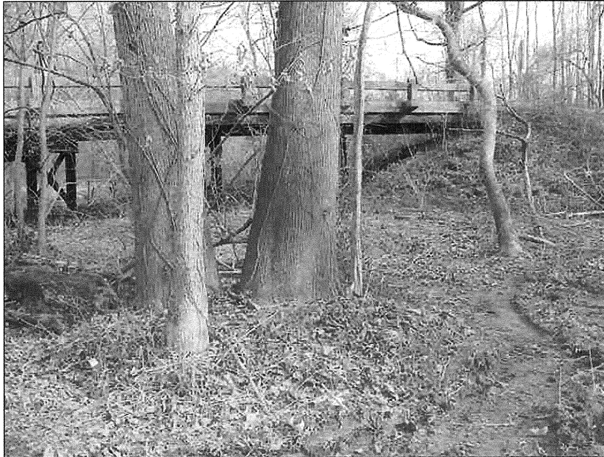
End Bent 1, looking from EB1A to EB1B.
