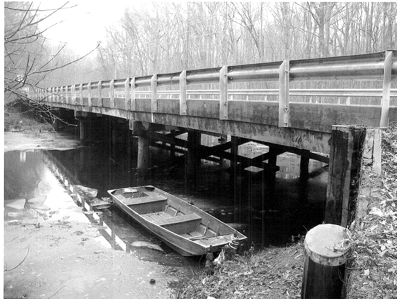
Looking northeast towards End Bent 2
