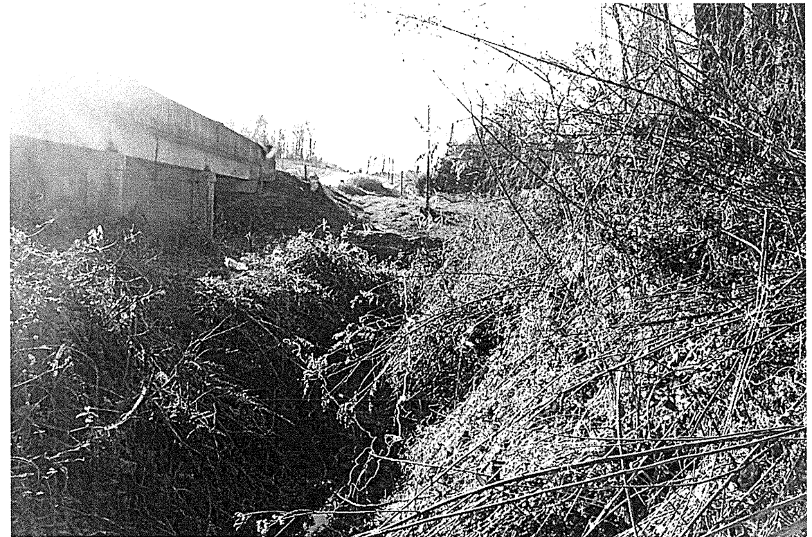
View Approximately 19' Left of -L- Looking Downstation from End Bent-2
