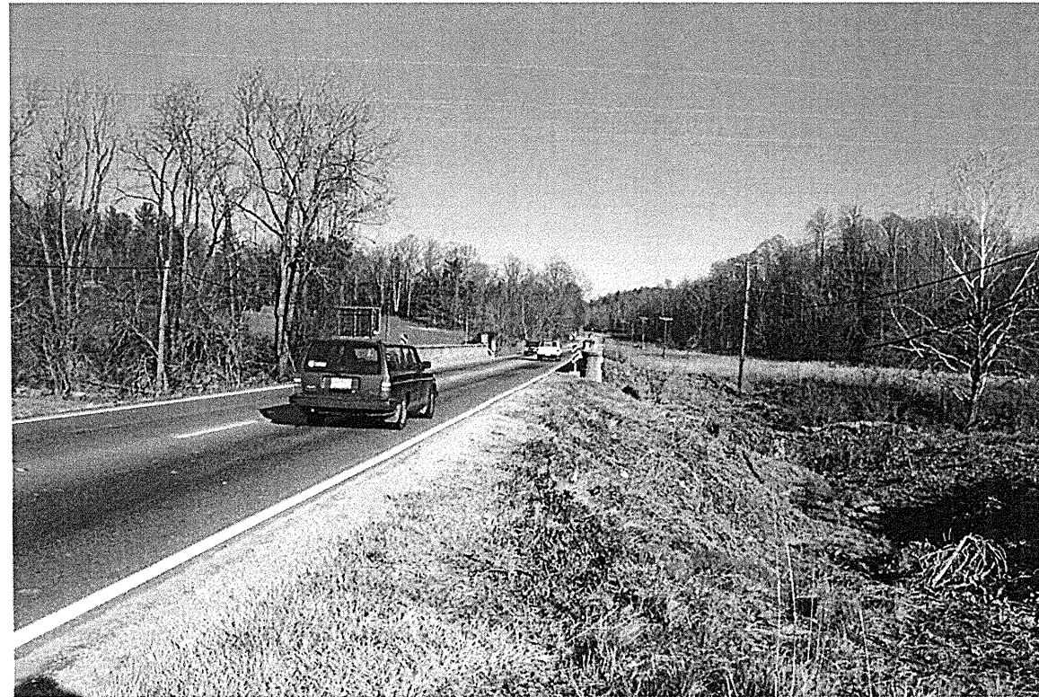
View of Existing Bridge Looking Upstation
