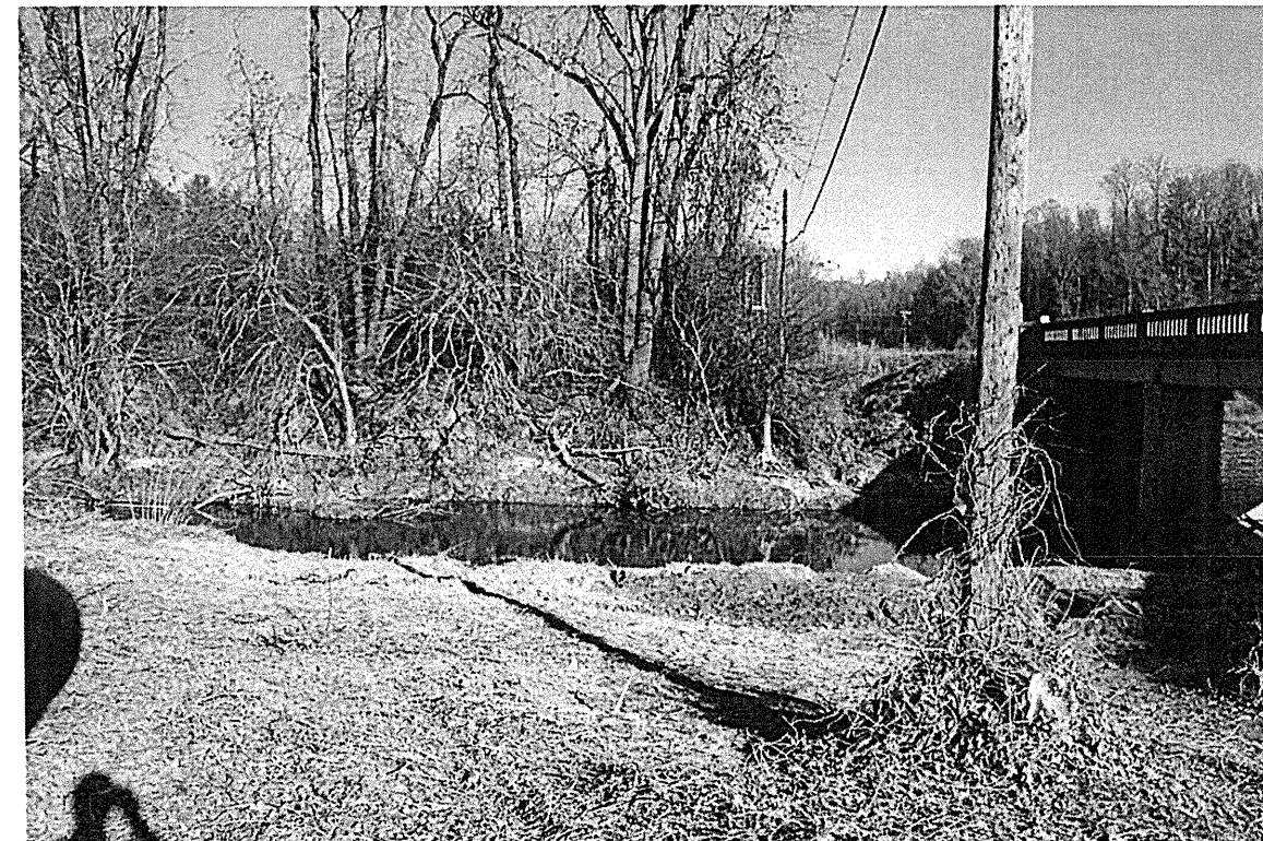
View Approximately 19' Left of -L- Looking Upstation from End Bent-1
