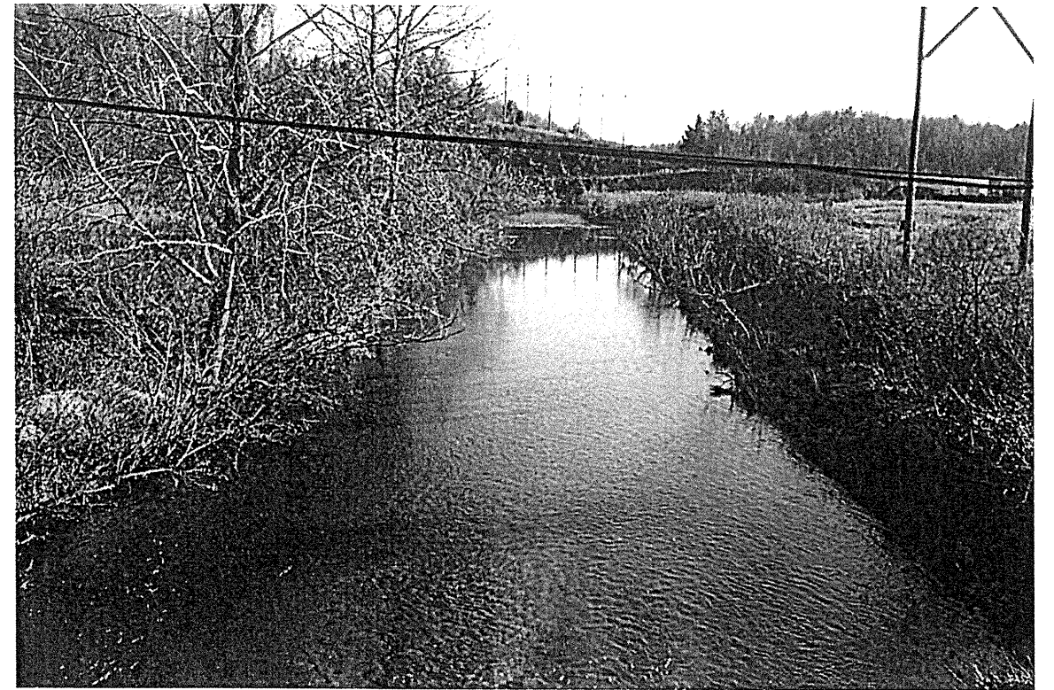
View Downstream from Existing Bridge
