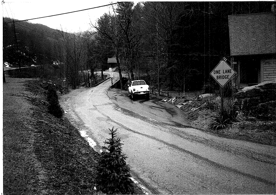
Bridge No. 94 on SR-1111. View looking west.
