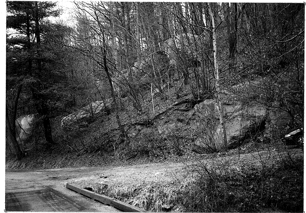
Site of proposed retaining wall. View looking West across proposed EB1.
