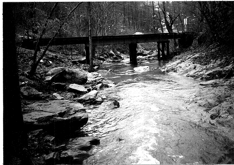
View down stream channel to Bridge No. 94.
