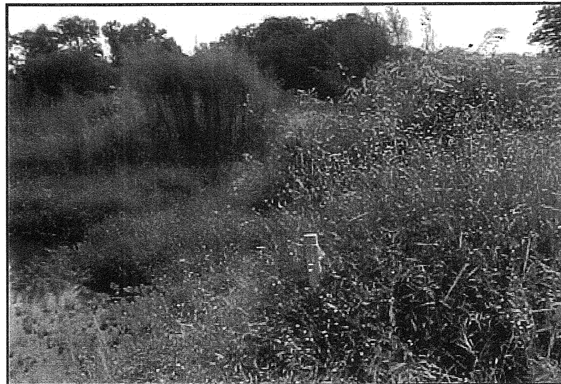
Photograph 14: View looking south along Left Lane Bent 3 from B3-A in foreground toward B3-B.
