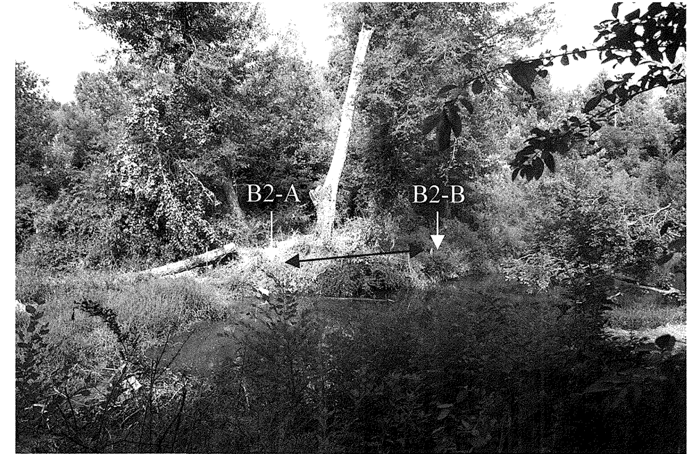
Looking West at Interior Bent 2
