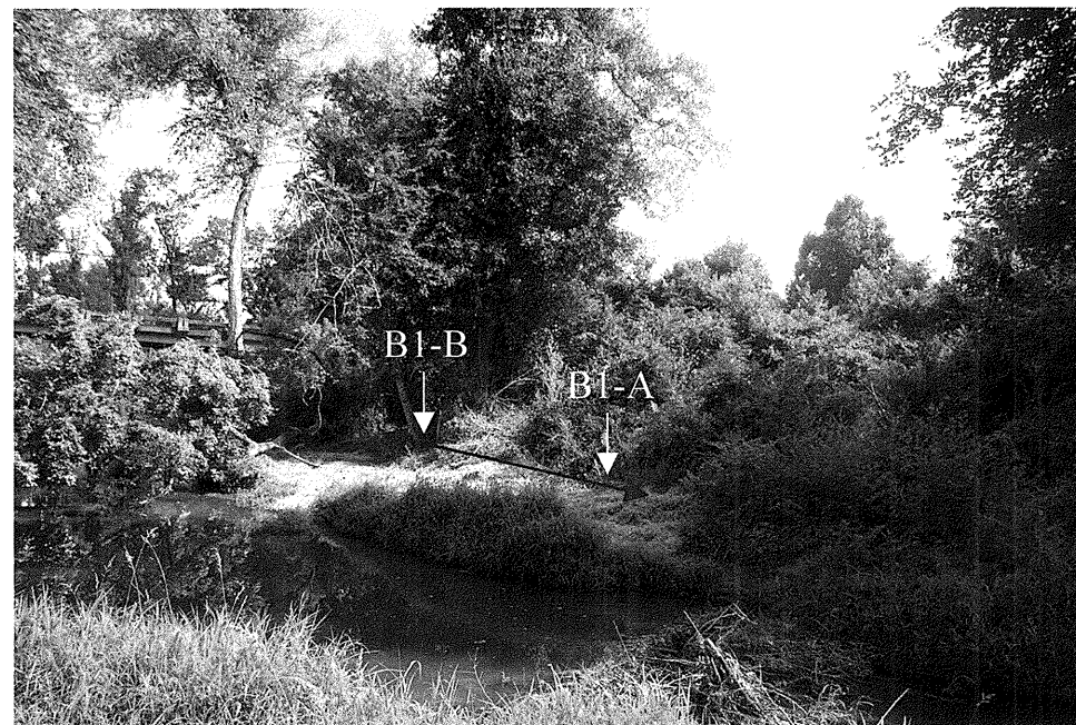
Looking North at Interior Bent 1
