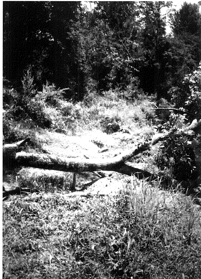
Looking southeast at the downstation side of the creek prior to restoration.
