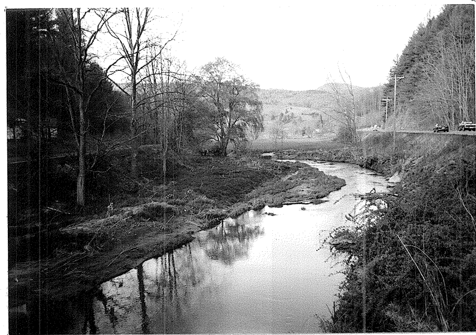
Figure 2. Looking downstream from Bridge 316 toward new bridge site on -L-. Willow tree is on Bent One. US 321 is on right side of photo.
