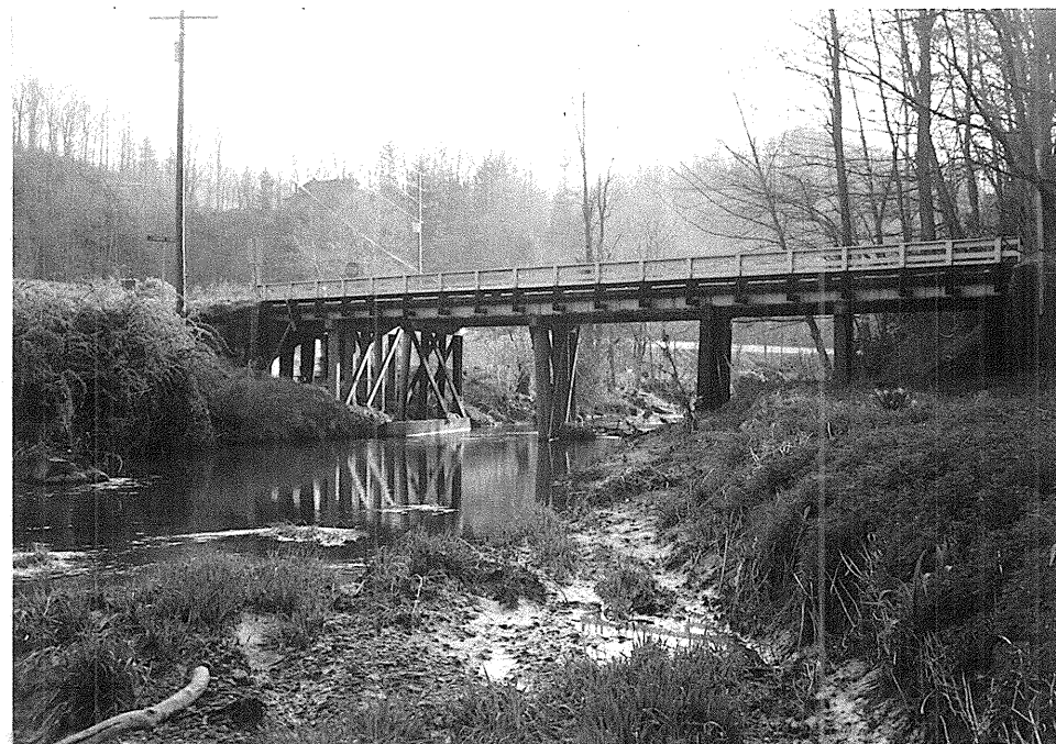
Figure 1. Bridge 316 on SR 1149. View looking upstream.
