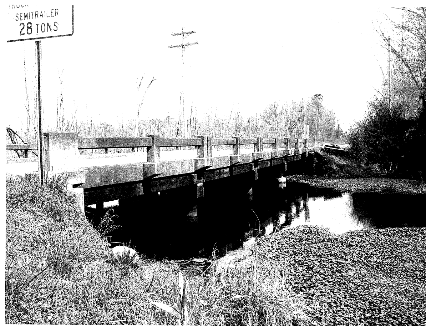
Looking east towards End Bent 2
