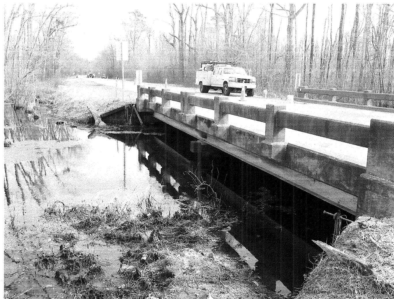
Looking east towards End Bent 2
