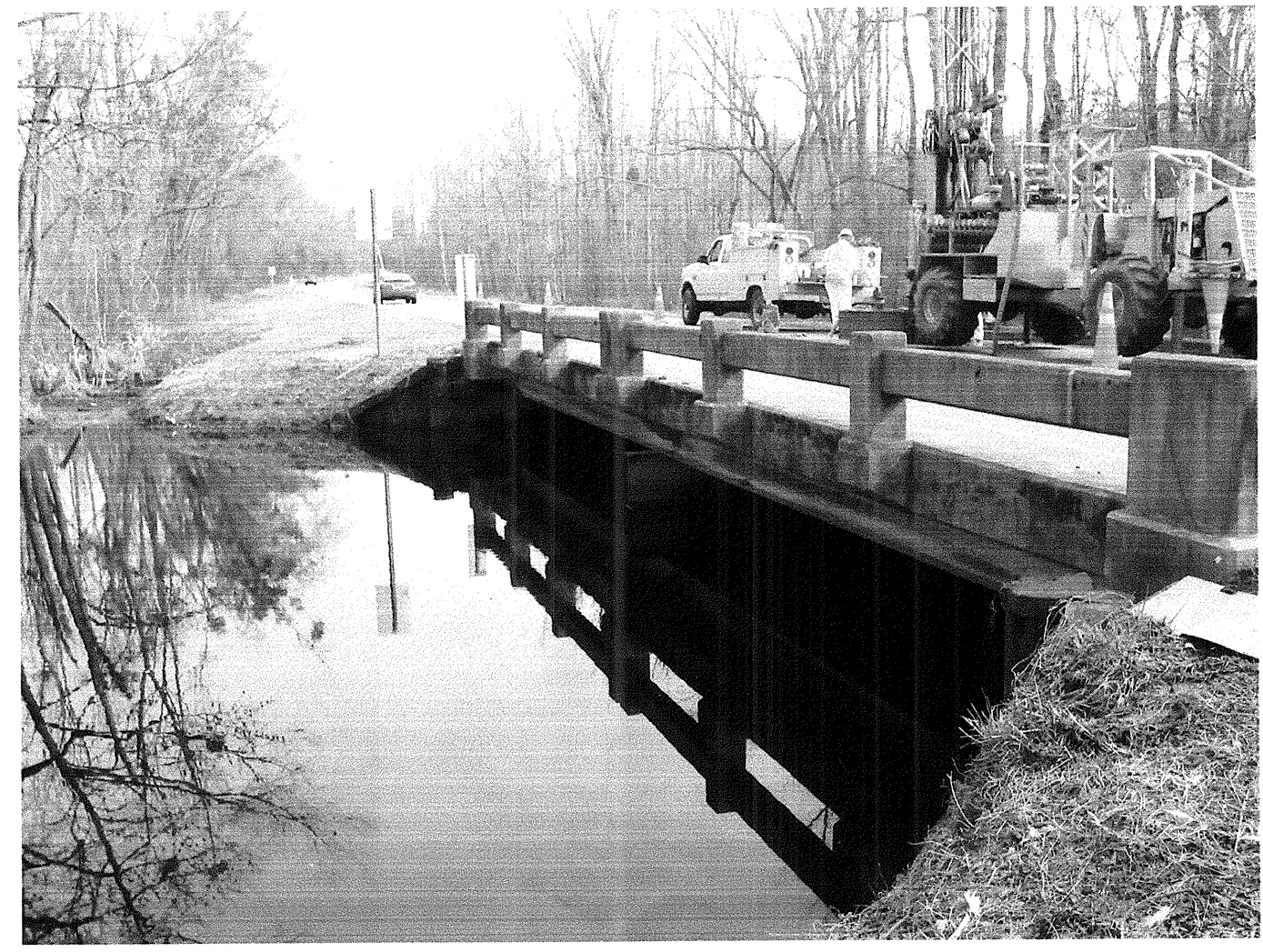
Looking east towards End Bent 2
