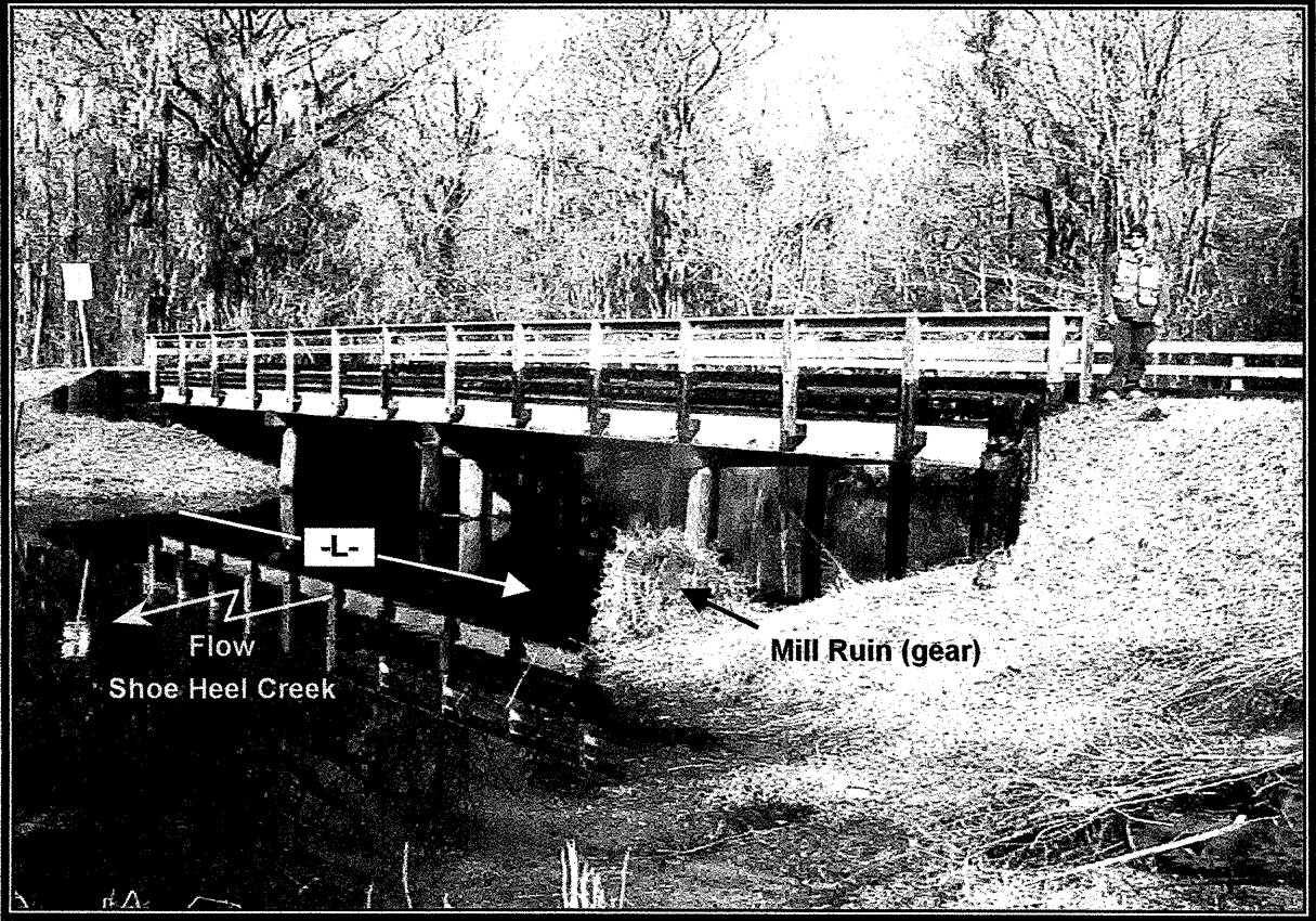
SITE PHOTOGRAPH - BRIDGE NO. 170, ROBESON COUNTY
