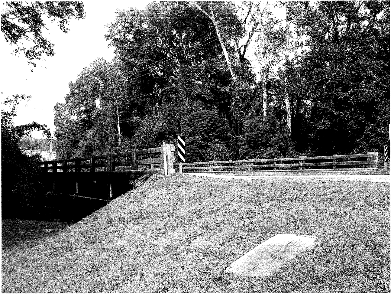
Looking west towards End Bent 1
