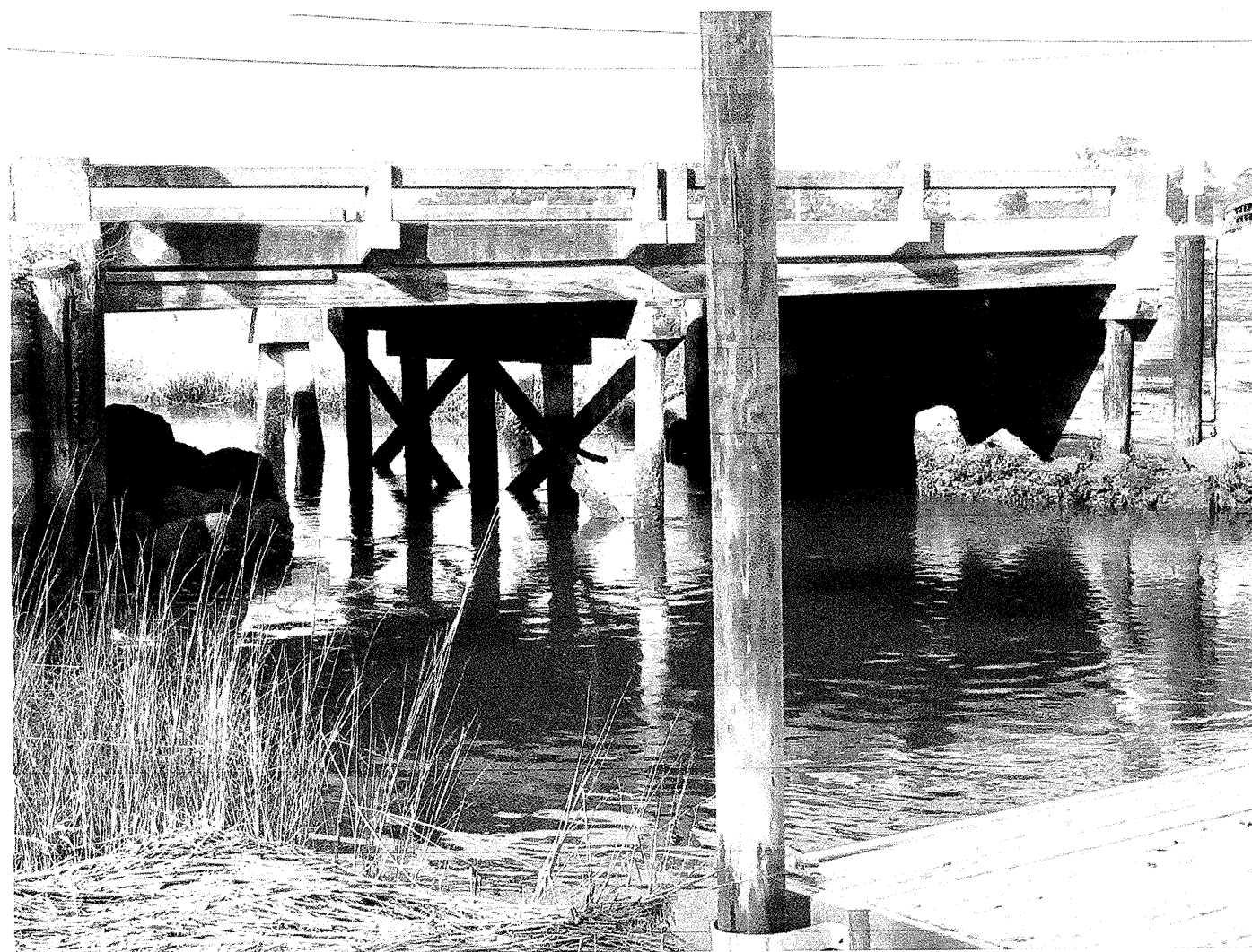
Looking north towards End Bent 2
