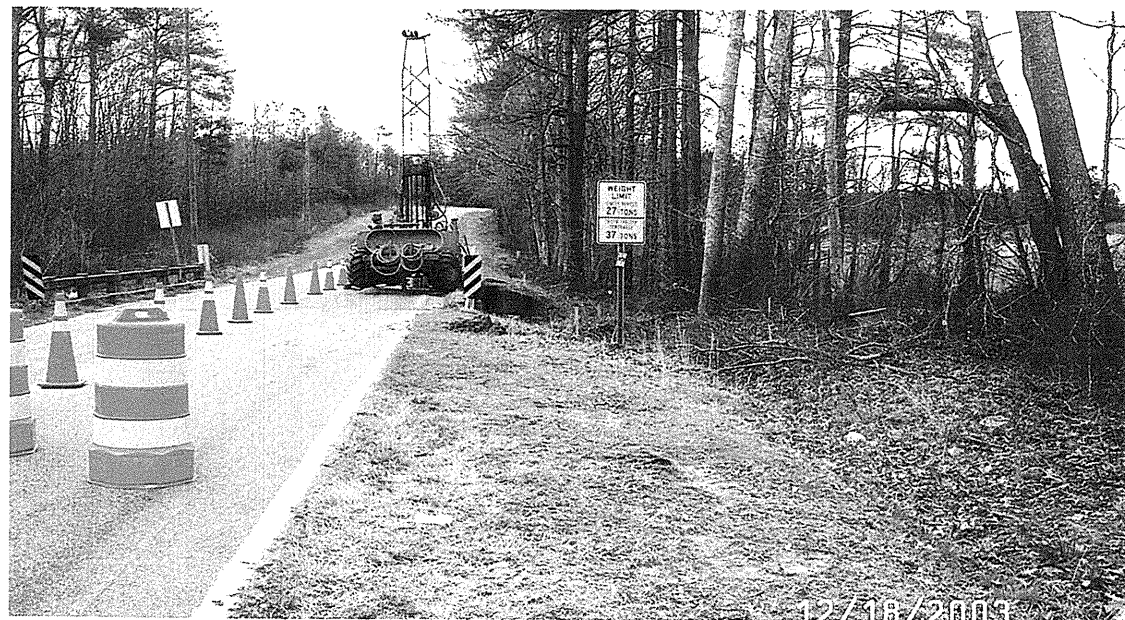
View along "A" Borings from End Bent 2 towards End Bent 1
