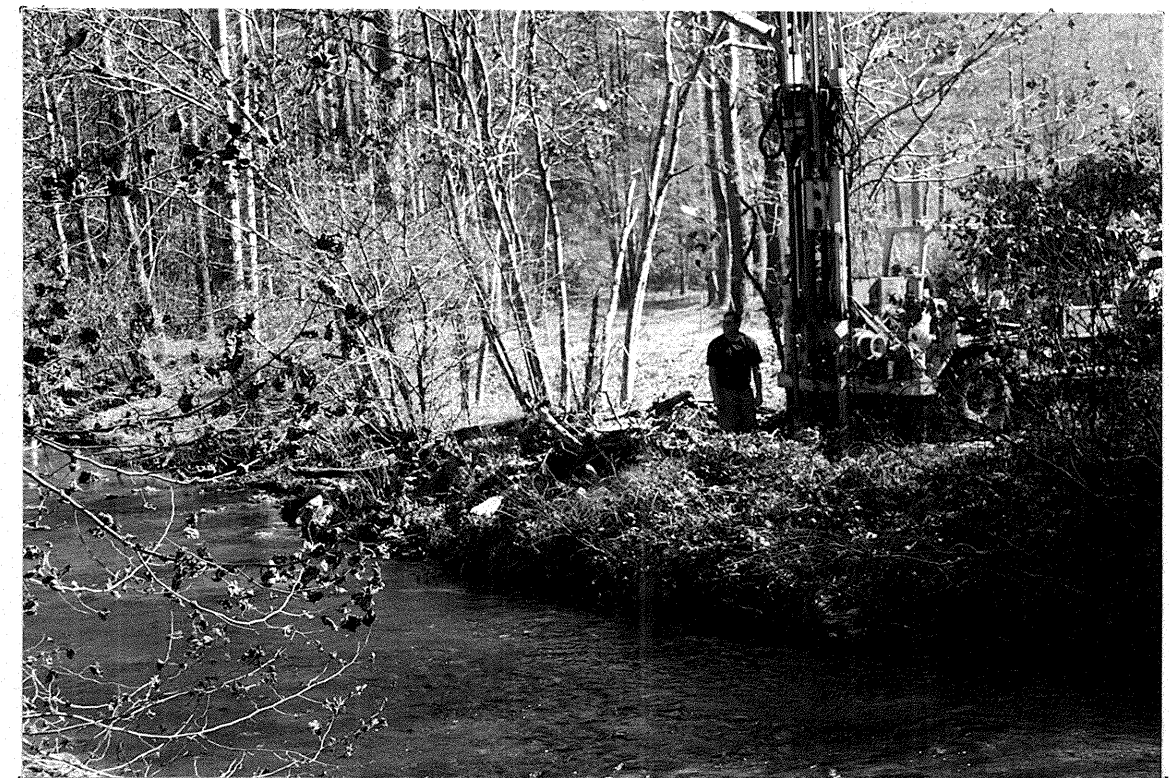
Drilling at Bent Two
