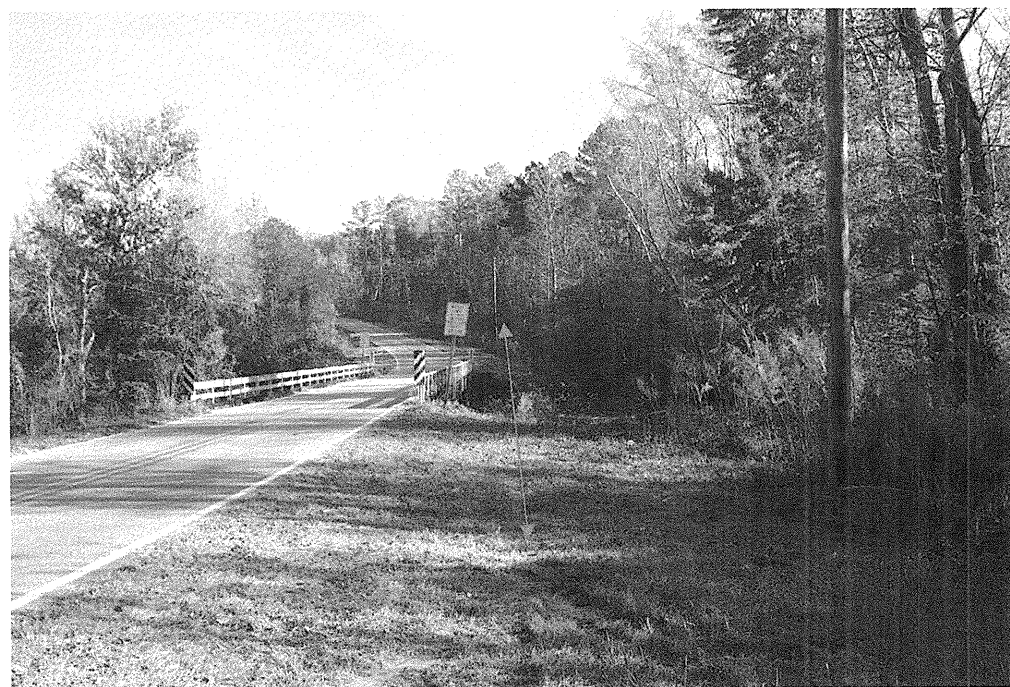
Photograph No. 5: Profile view looking south from End Bent 1.
