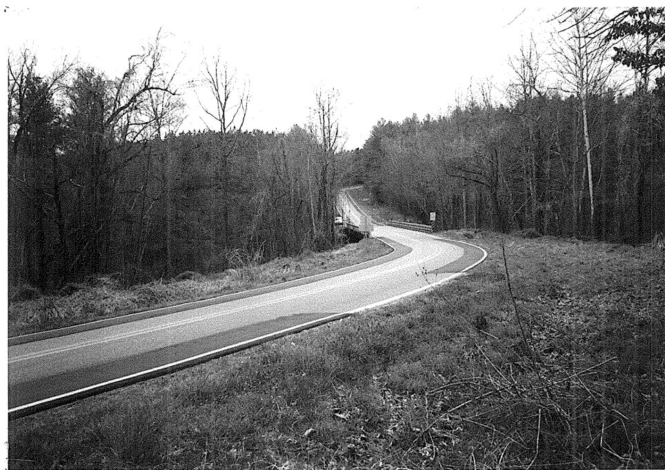
Figure 2: Looking forward from Station 11+00. New alignment is on right side of photo.
