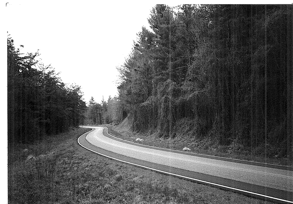
Figure 4: Looking forward to end of project from Station 22+00.
