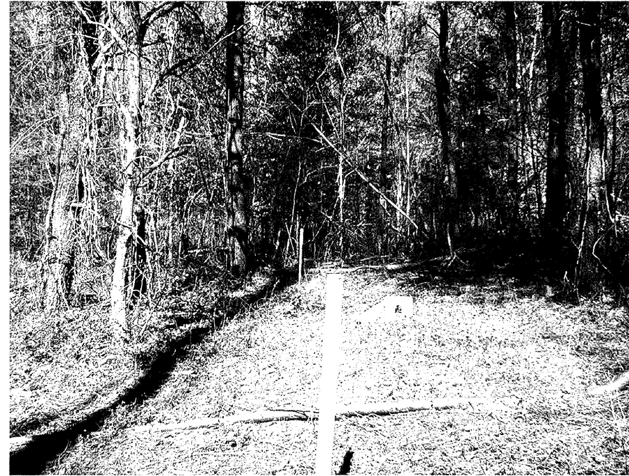
Looking Left to Right along End Bent-1
