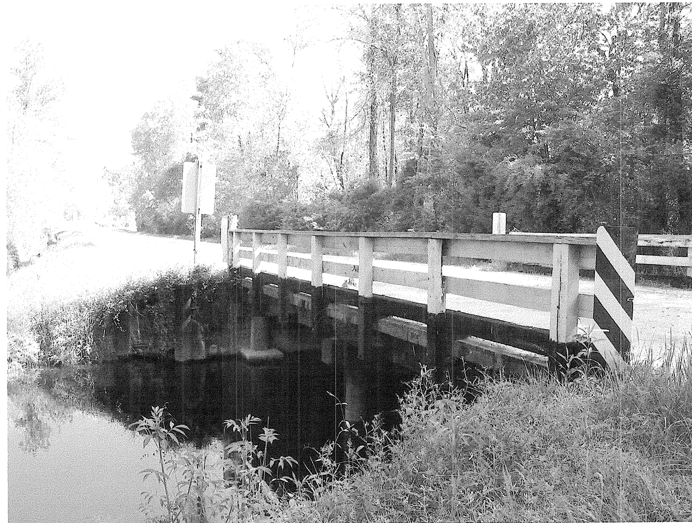
Looking north towards End Bent 2
