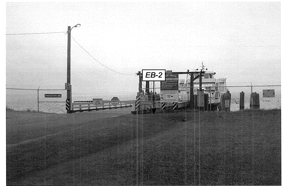
Photograph 8: View to Southwest showing approximate location of boring EB-2 at the Knotts Island Ferry Dock site.
