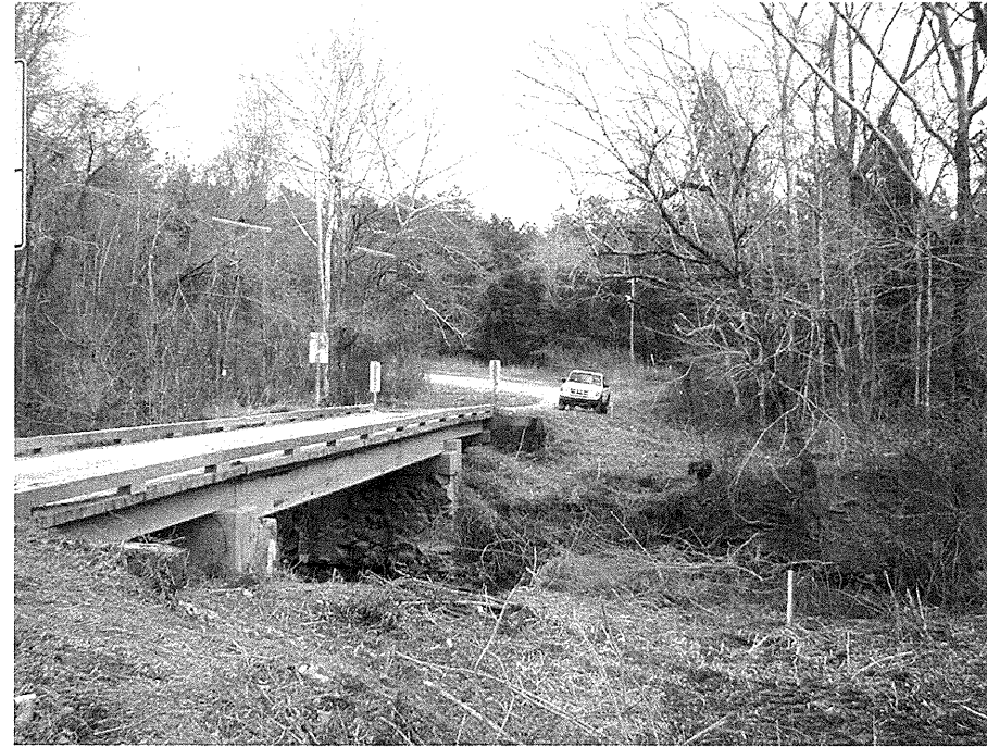
Looking Increasing Station along -L-
