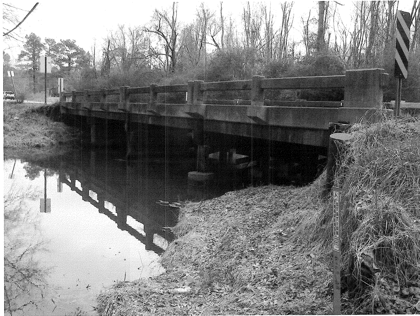
Looking southeast towards End Bent 2
